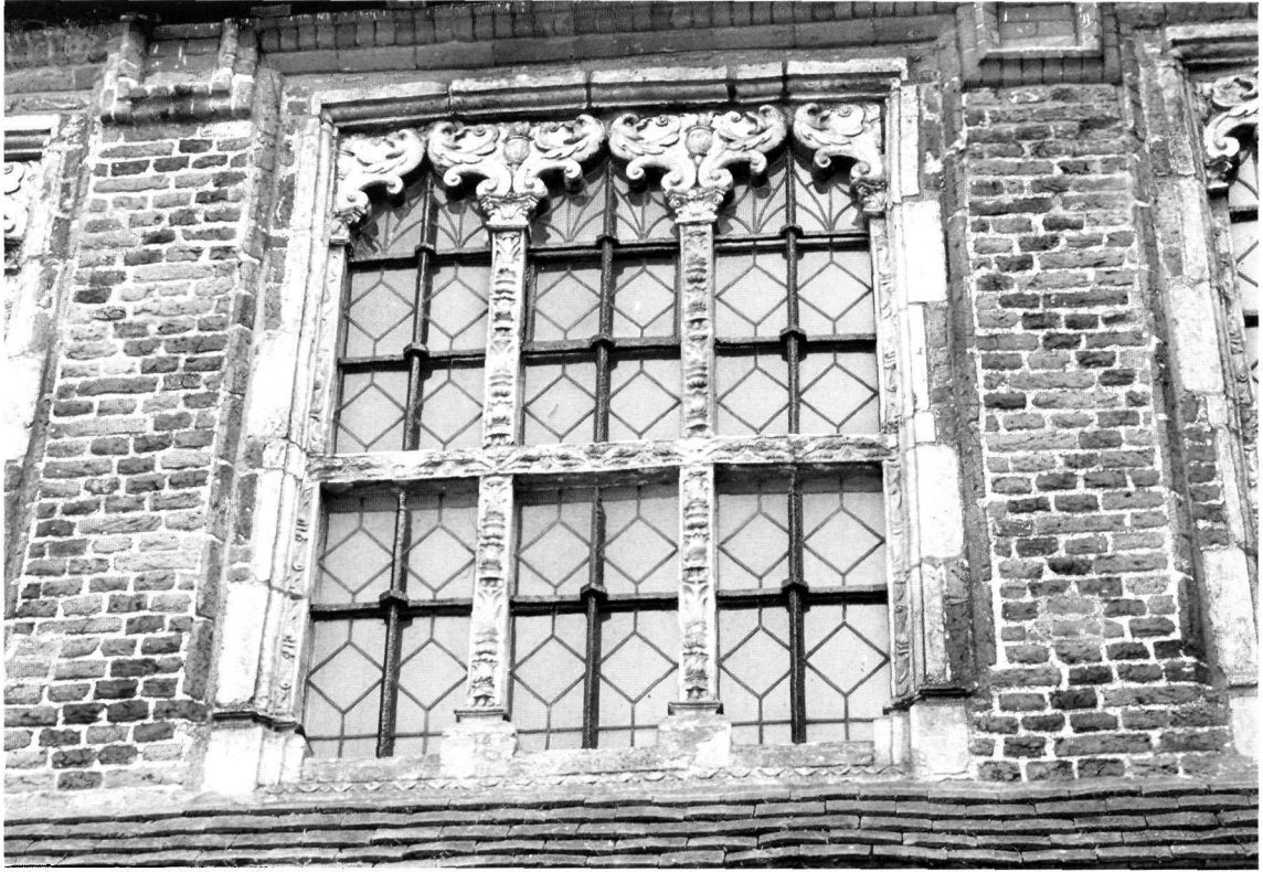
Fig 22. View of a gatehouse window at Layer Marney, Essex, showing the use of early 16th-century terracotta decoration (Photo by Gordon Malcolm)
