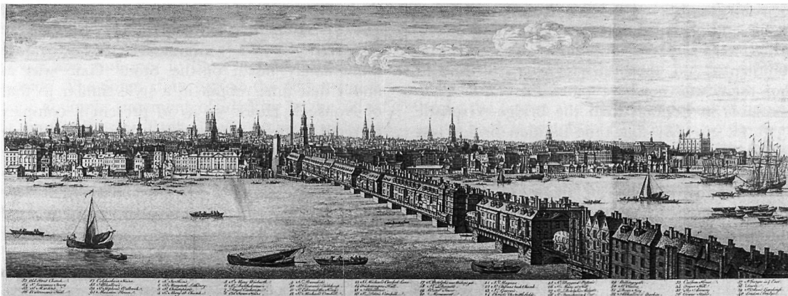
Fig 6. London Bridge from the south-west c.1748. Drawn and engraved by S and N Buck, published 1749. The bridge is once more almost entirely occupied by houses, which from this time onwards were progressively removed as the structure was 'improved'. (Copyright: Guildhall Library, Corporation of London)
