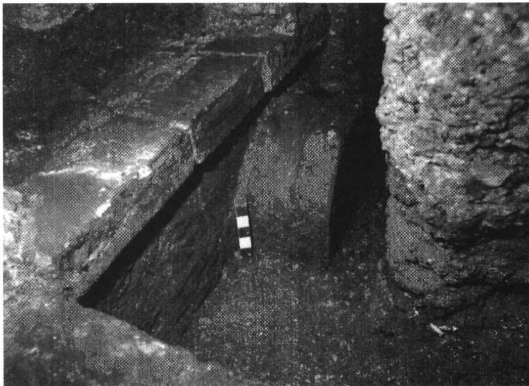
Fig 12. Phase X repairs to wall and possible mooring-point
