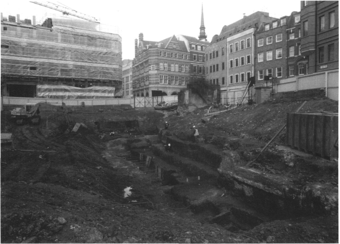
Fig 2. General photograph of the site, looking to the north-east
