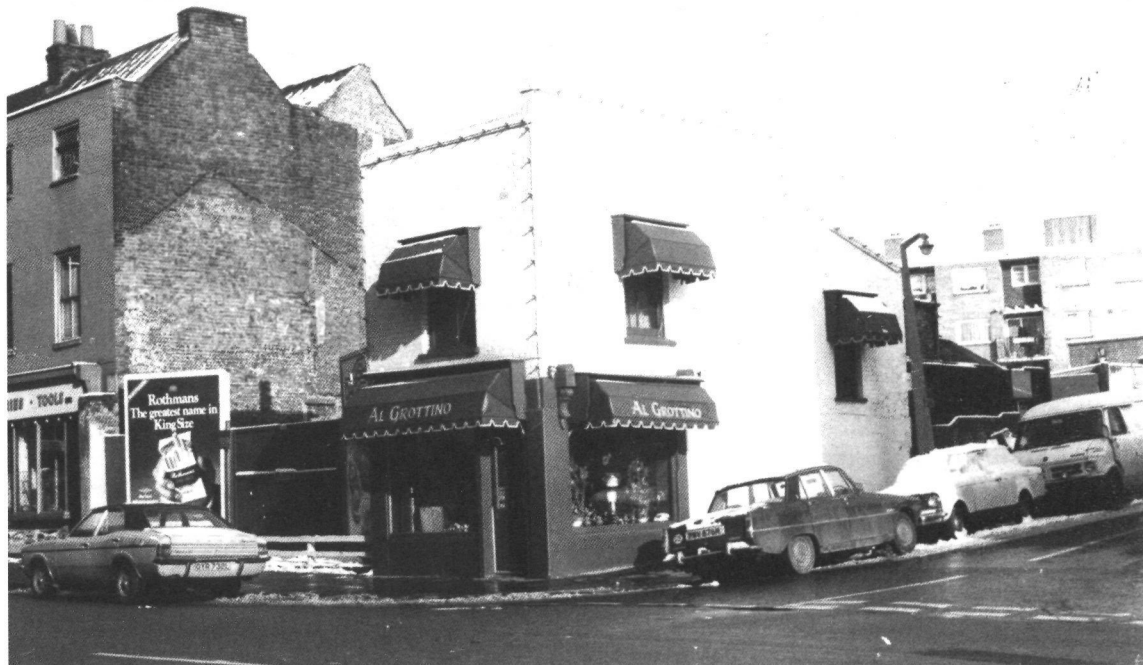
Fig 12. View showing roof scars of No. 31 Fulham High Street, No. 35 is shown standing, 1979
