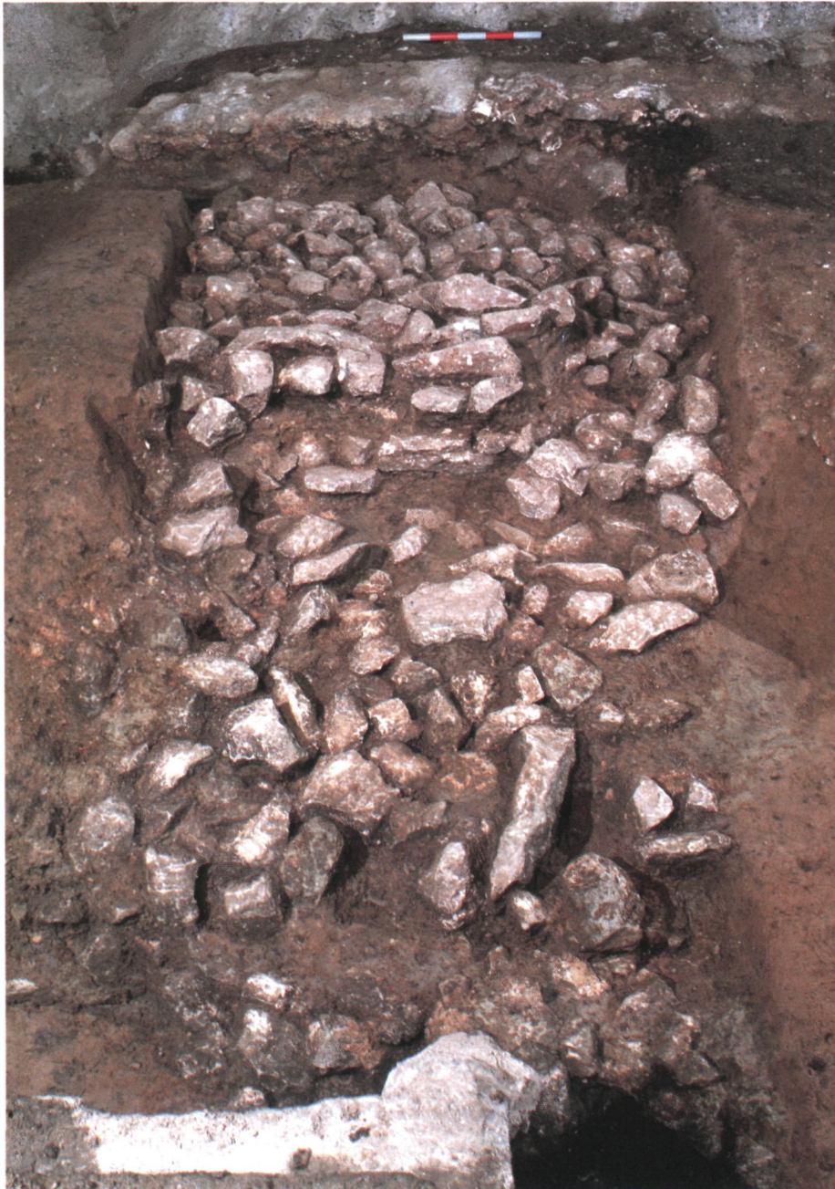
Fig 4. Foundations of south wall of Cripplegate fort (Structure 1), looking east (0.50m scale)
