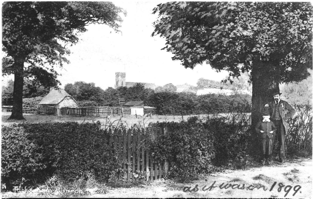
Fig 10. It's very difficult to find a photograph of a laburnum leaning on railings; but here are some railings leaned on by a profusion of vegetation, in a Lordship Lane, Tottenham scene unrecognisable today
