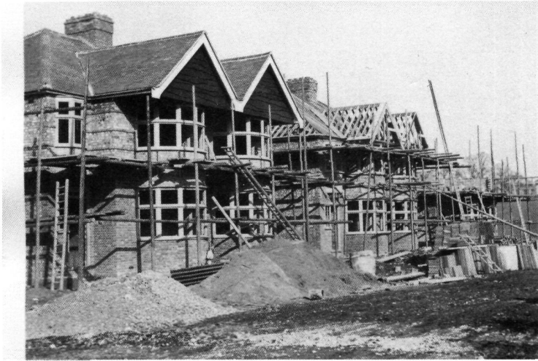
Fig 49. New houses going up somewhere in Wembley, 1920s
