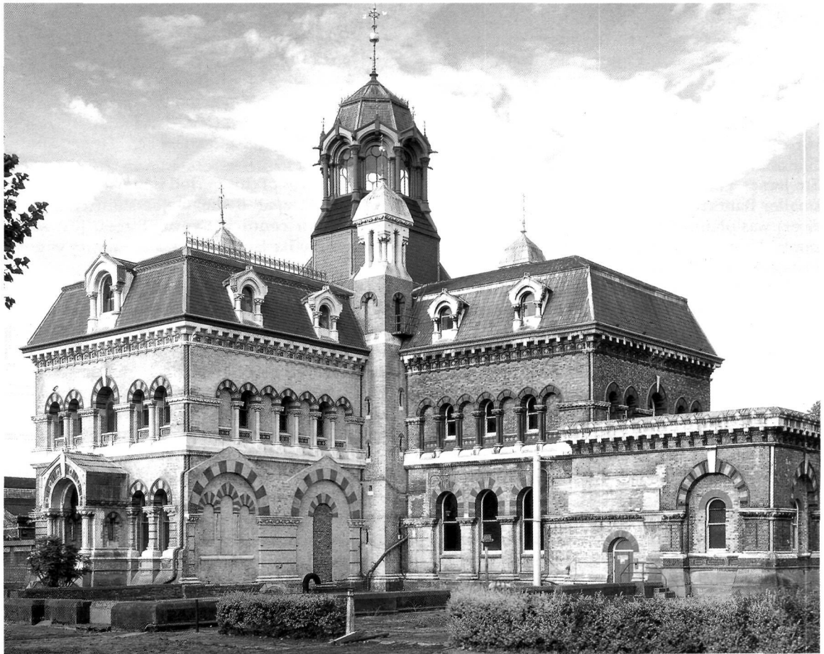
Fig 4. The Pumping Station at Abbey Mills, Stratford
