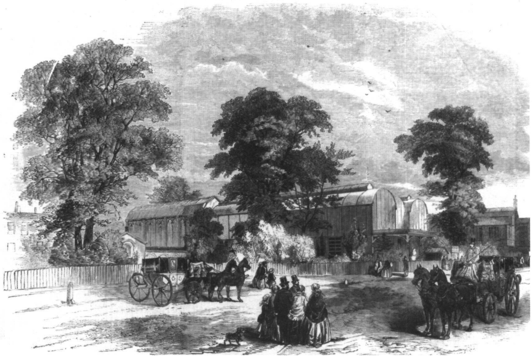
Fig 2. The South Kensington Museum in 1857: in a rural setting, and serving the carriage trade (Illustrated London News, 27 June 1857; by courtesy of the Trustees of the Victoria and Albert Museum)
