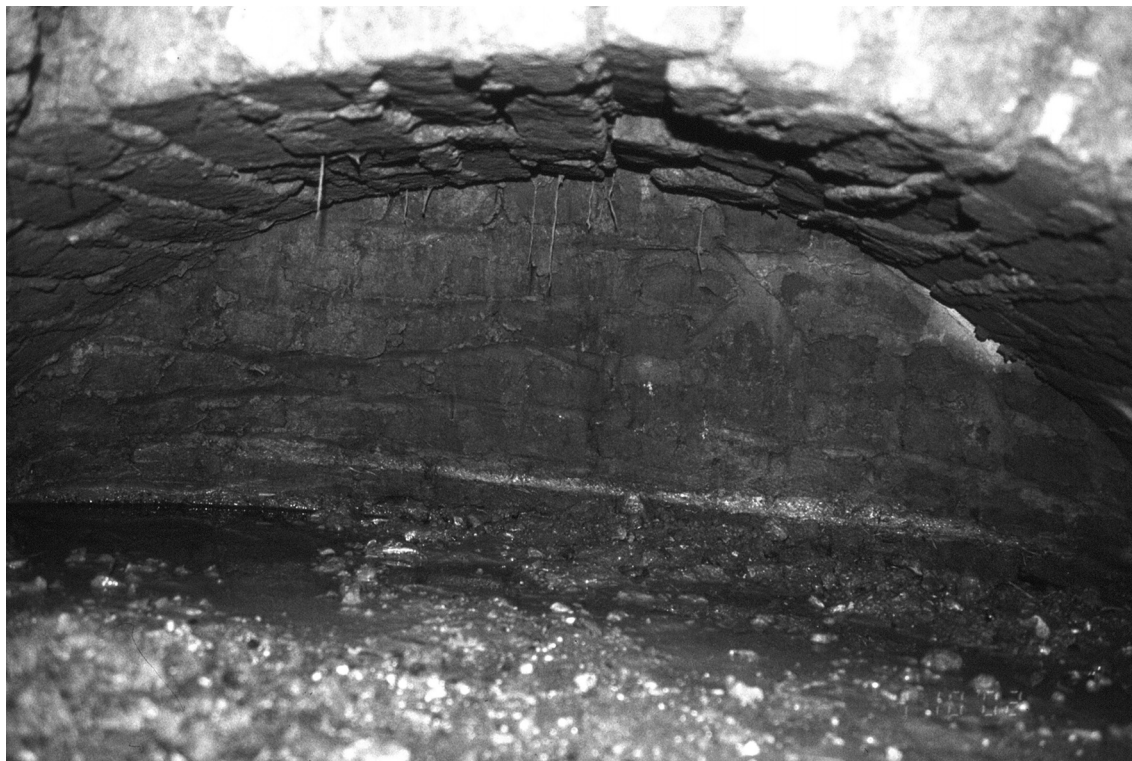
Fig 6a. East view of ha-ha wall in Trench 2
