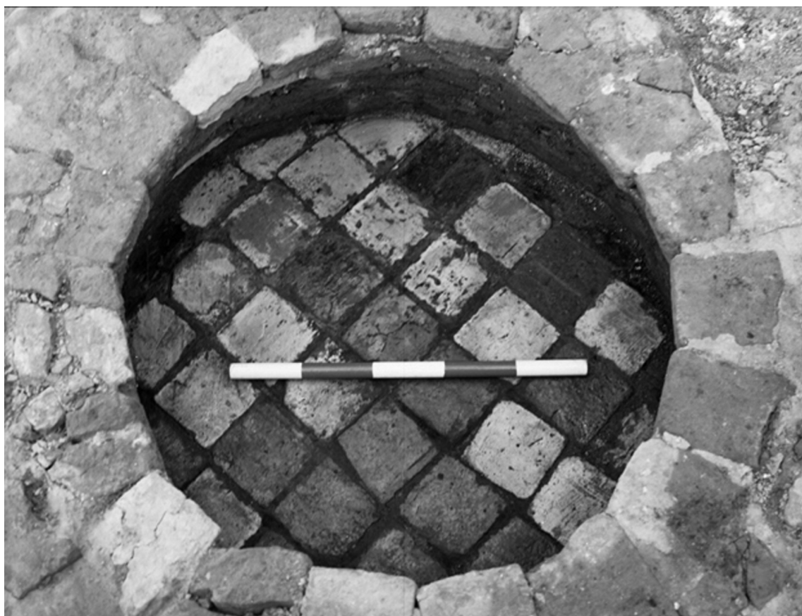
Fig 9. Site 1: 'Beehive'-shaped brick structure
