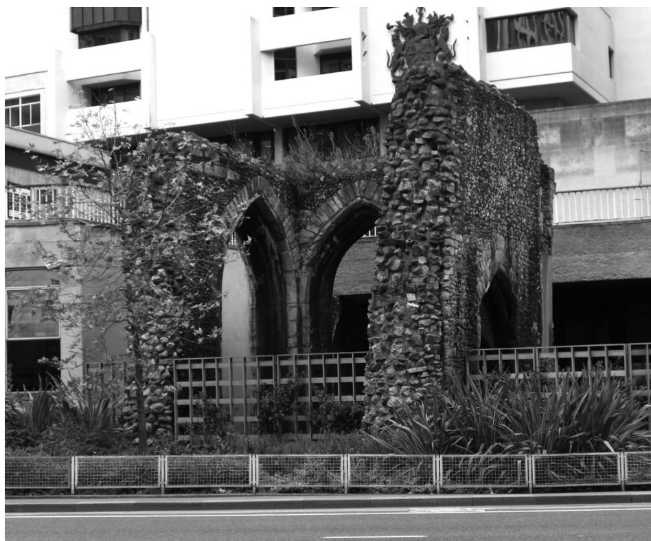
Fig 2. The base of the tower of St Alphage church on London Wall, previously the church of Elsyngspital
