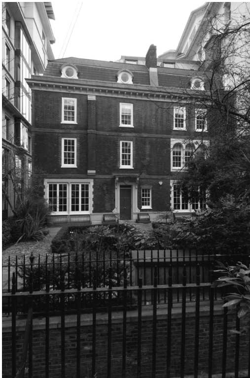
Fig 8. View of the north façade of the house, looking over the former churchyard of St Laurence Pountney, now the garden of the house; the six tall and narrow window openings and the string courses are original features of the house of c.1670
