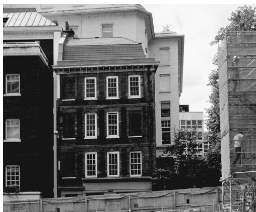
Fig 7. View of the east façade of the house, fronting onto Laurence Pountney Lane (the view no longer exists: the photograph was taken in 2003 in a brief window of opportunity between the demolition of one large building on Arthur Street and the construction of its successor)
