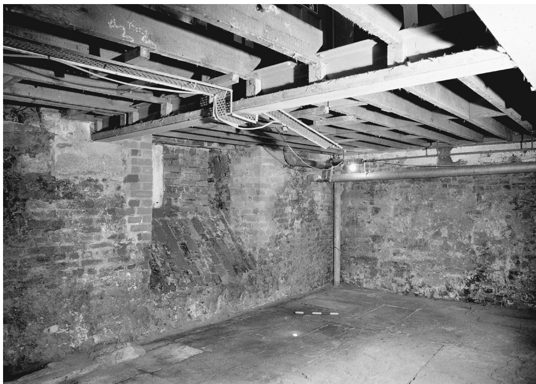
Fig 2. View of the medieval walls preserved in the east and south walls of the basement of the 17th-century house (with 17th- and 20th-century brick alterations) (1.0m scale)
