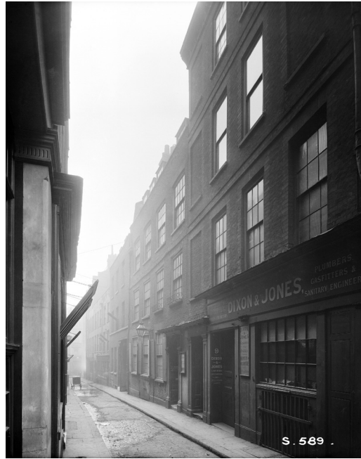
Fig 14. Photograph of the 1860s or 1870s looking south-west down Laurence Pountney Lane, showing the 18th-century shopfront, originally of the hop merchant Benjamin Winthorp ('Dixon and Jones'; NMR, DD75/15)
