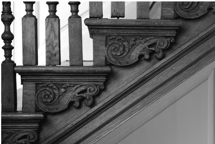
Fig 12. Detail of the staircase of c.1730: the flower scrolls on the string
