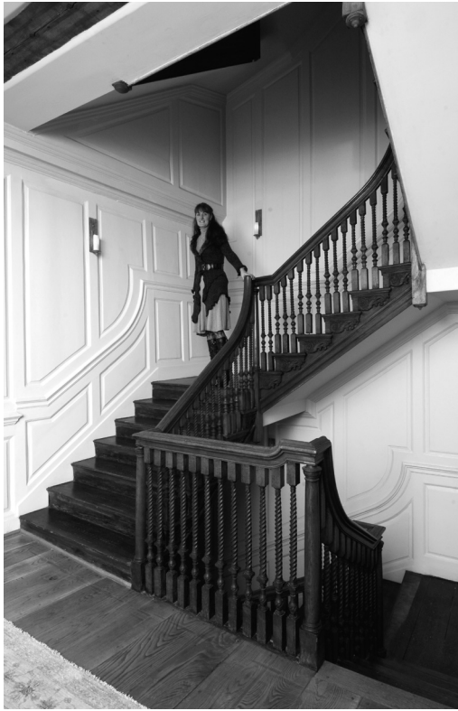
Fig 11. View of the staircase of c.1730 after restoration
