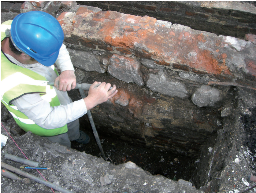
Fig 8. Auguring within the cellar, east facing
