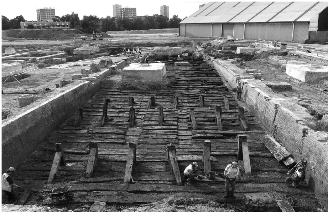
Fig 3. The 19th-century slipway in Area 4 of the MOLA excavation of the Deptford Royal Naval Dockyard, view looking south-west. The vertical and raking timbers post-date the dockyard (Photo: MOLA)
