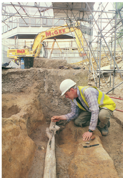
Fig 19. Lead pipe forming part of conduit under excavation on Site C, with repair to pipe in foreground
