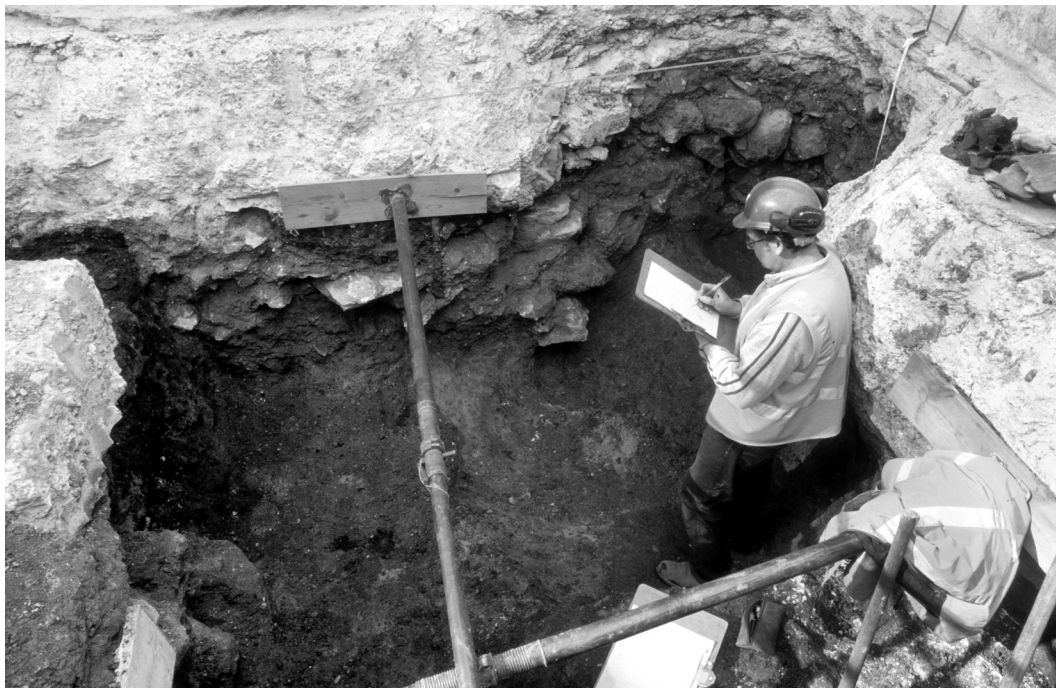
Fig 21. A section through the foundations of Building 11 as recorded in the south-east corner of site
