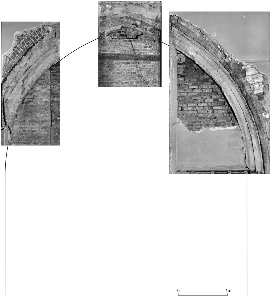
Fig 7. Montage of photographs of 1929 (with corrected perspectives) showing an arcade arch dividing the choir of Austin Friars from the parish church of St Peter the Poor, looking south towards St Peter (scale c.1:40) (note that the middle photograph is the opposite viewpoint but has been reversed for consistency; English Heritage Archive, OP 15755, 15758 and 15760)
