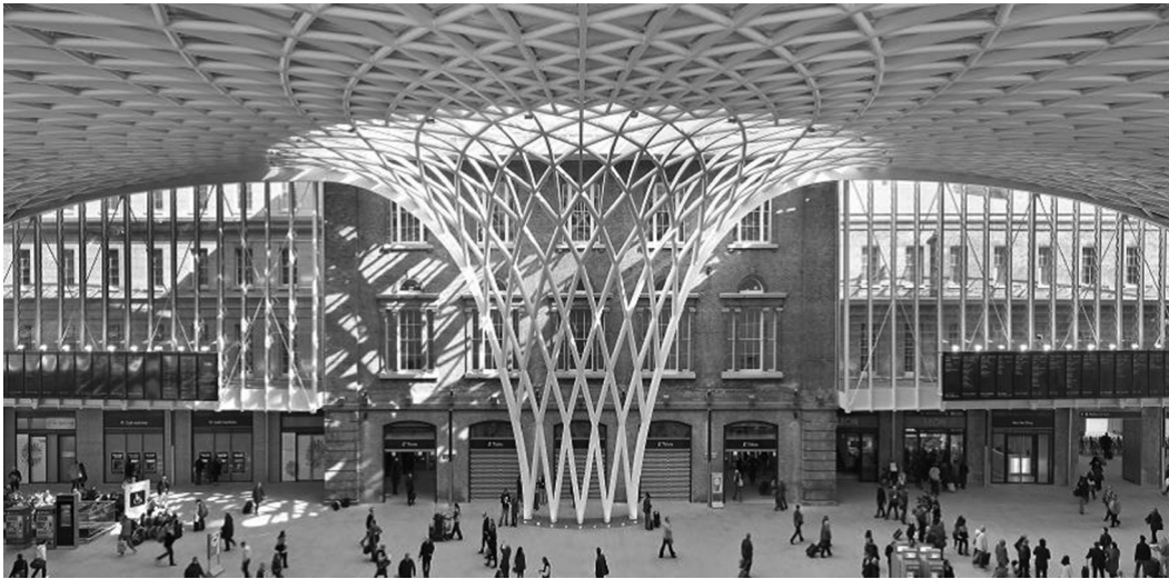
Fig 8. The new concourse at King's Cross Station (Photo: Hufton & Crow/John McAslan & Partners)
