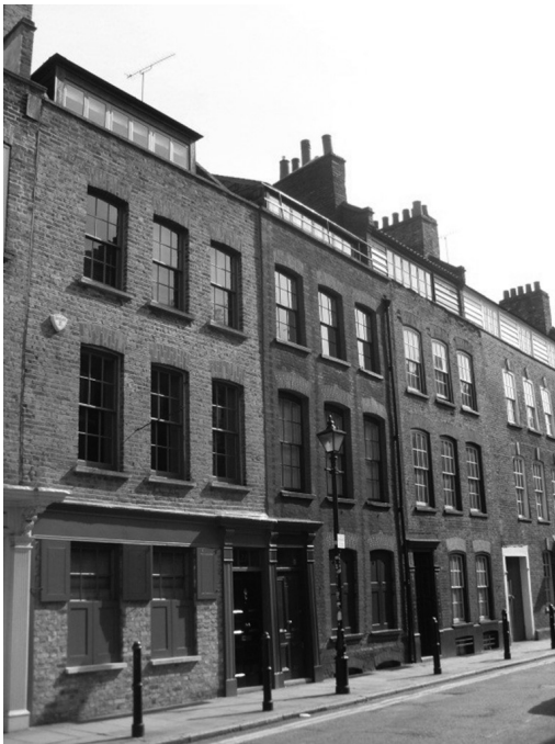
Fig 3. Three-bay Georgian terraced houses in Fournier Street (Photo: Alec Forshaw)
