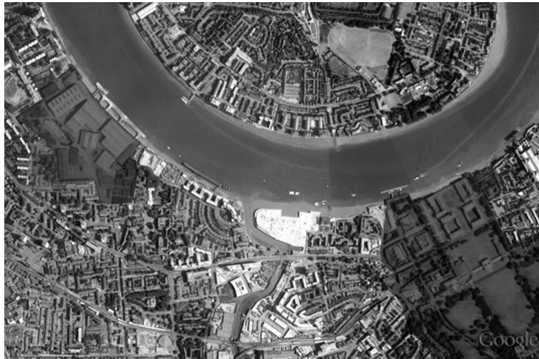
Fig 6. Aerial photograph highlighted to show Convoys Wharf (left) and the Maritime Greenwich World Heritage Site (right) (Photo: Alan Baxter Associates)
