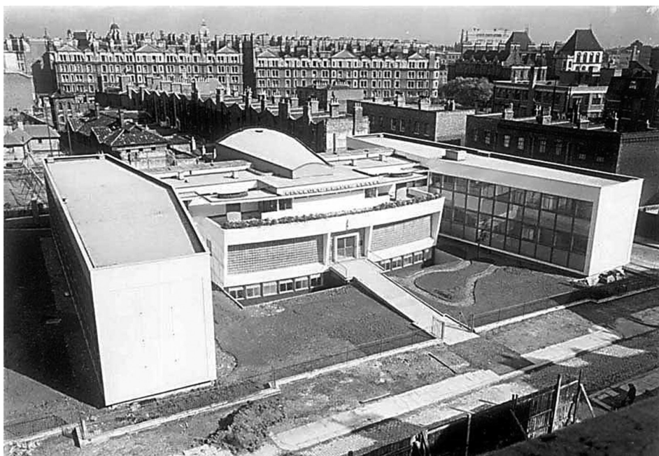
Fig 5. The Finsbury Health Centre in 1938 (Photo: Lubetkin, courtesy of John Allan)
