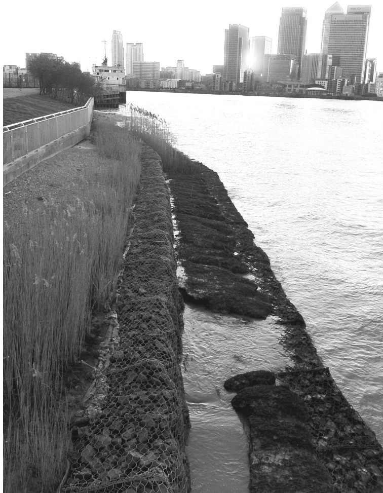
Fig 3. Environmental Agency 'inter-tidal terracing' at Greenwich Peninsula, 2011. Background: Canary Wharf, scene of conflicts between central government and local groups over dockland development in the 1970s and 80. (Photo: author)
