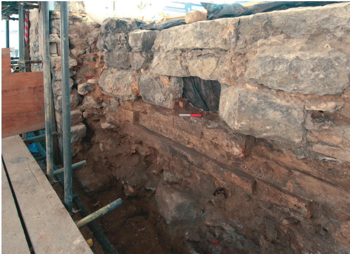
Fig 3. Moat wall (S1) dismantled showing facing associated with the Proof House (B1), looking south-east (0.2m scale)
