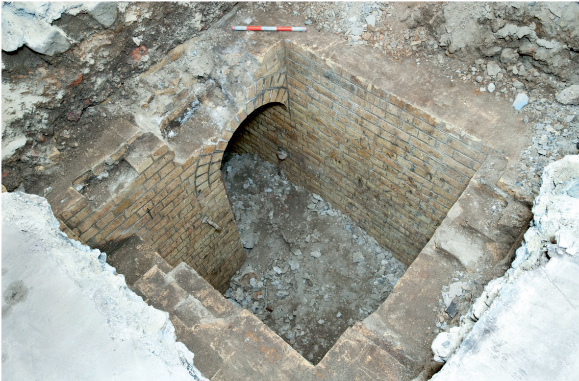
Fig 12. Brick-built chamber (S5) with tunnel entrance, looking north-west (0.5m scale)
