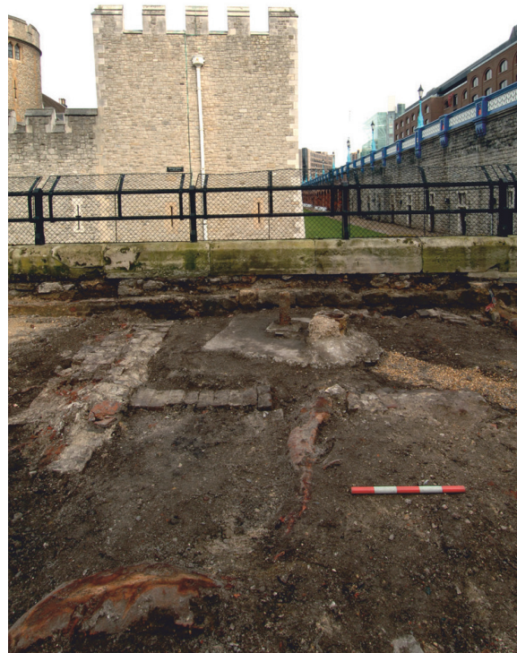
Fig 11. Walls of Building 7 built against the moat wall (S1), with Develin Tower in the background, looking north (0.5m scale)
