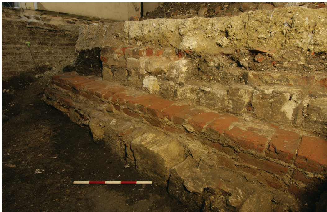
Fig 13. Masonry walling [171] over brickwork [172], built on wider masonry foundation [173] in Room B60, facing south (0.5m scale)
