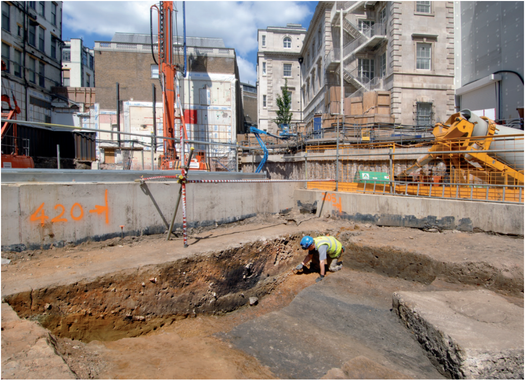
Fig 8. The period 5 ditch (S1) under excavation, including the east-facing section, looking north-west
