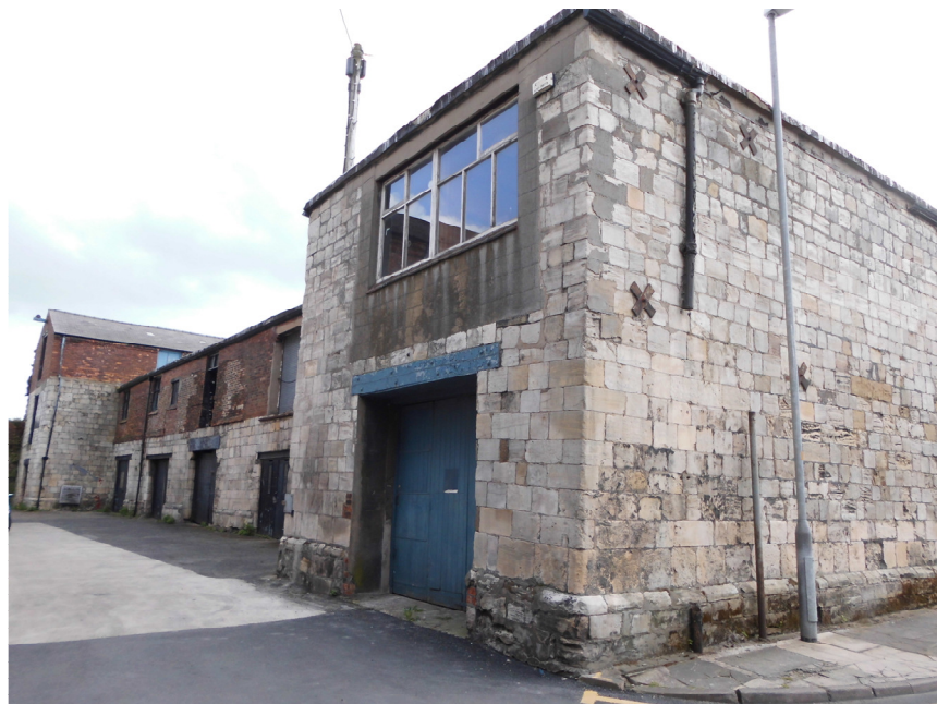
Staith Warehouse, North East Facing
