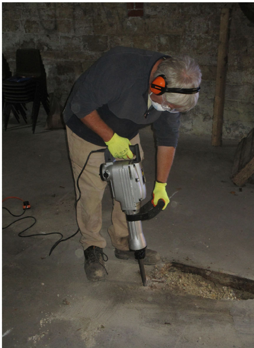
Dr Jon Kenny using power drill to open Trench 2
