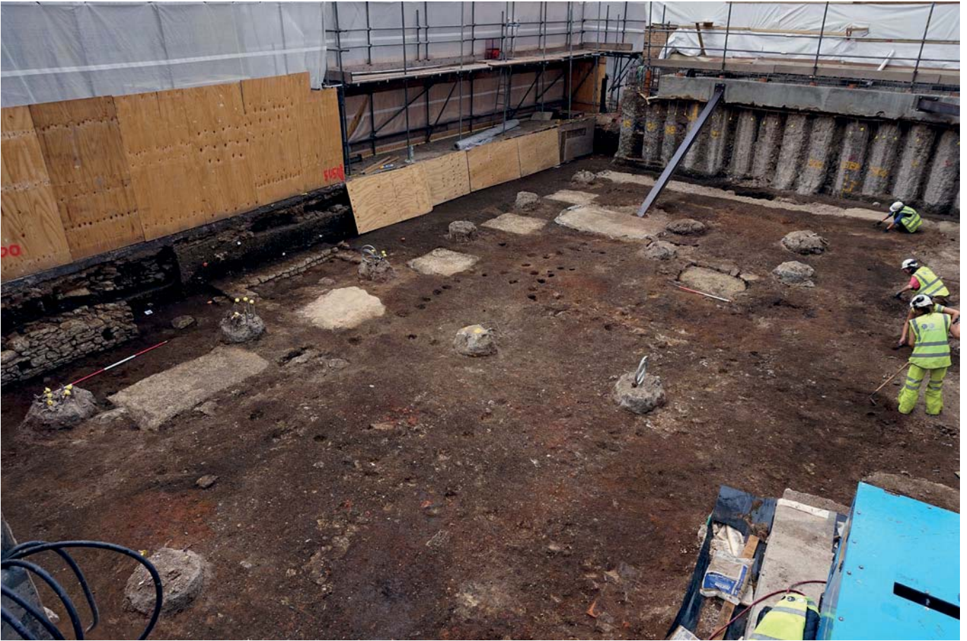
Figure 12: Area 4 after removal of basement slab showing unexcavated levels, Phase 6 stone-lined latrine 4073, looking SW
