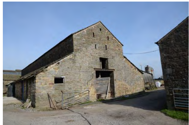
Plate 17 Southeast elevation of the barn
