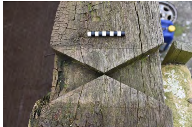
Plate 20 Upper part of wall plate showing notches for tie beam
