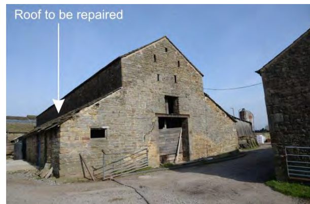
Plate 3 Southeast elevation of the barn
