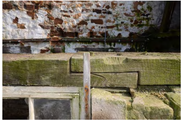
Plate 19 Wall plate towards the north end of the southwest outshut
