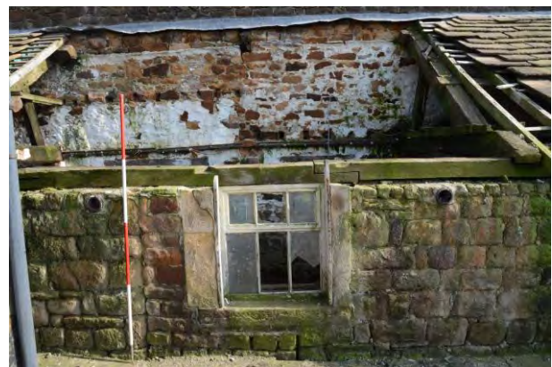
Plate 15 Window inserted in doorway, southwest elevation
