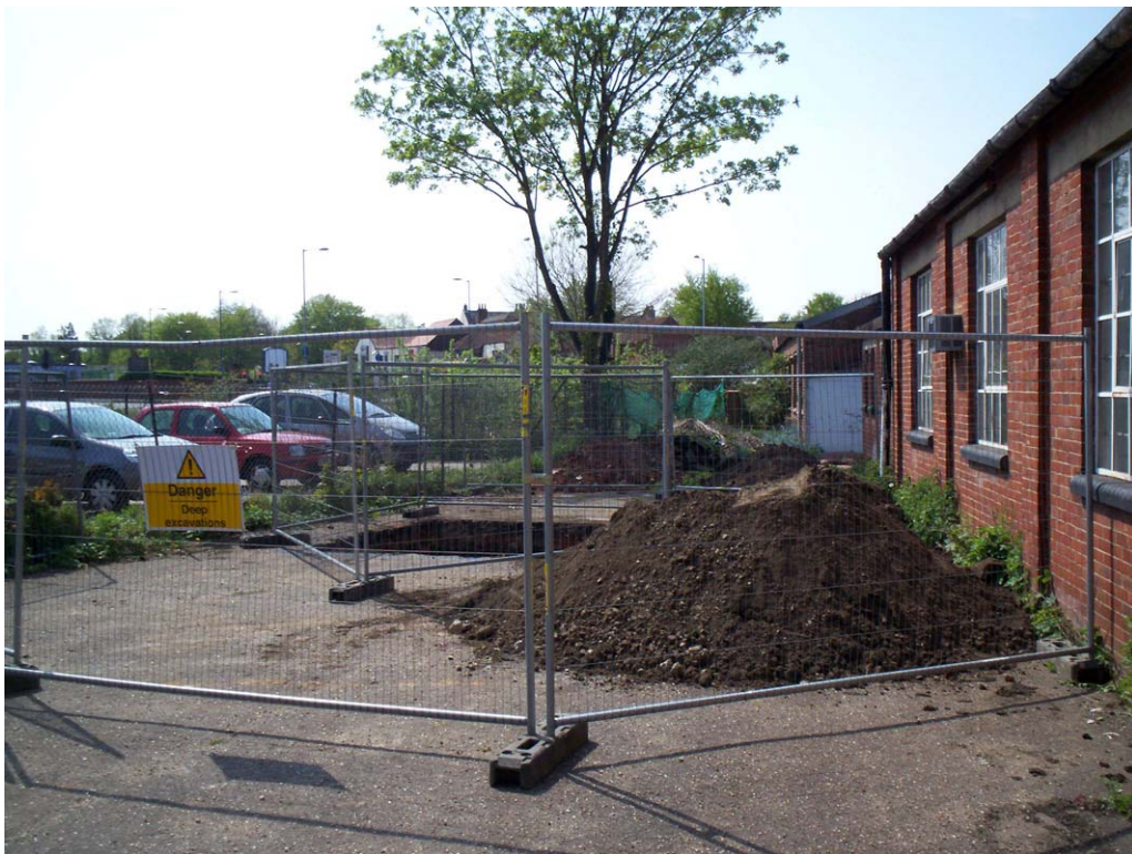
Plate 1. Trench 1, location, looking west
