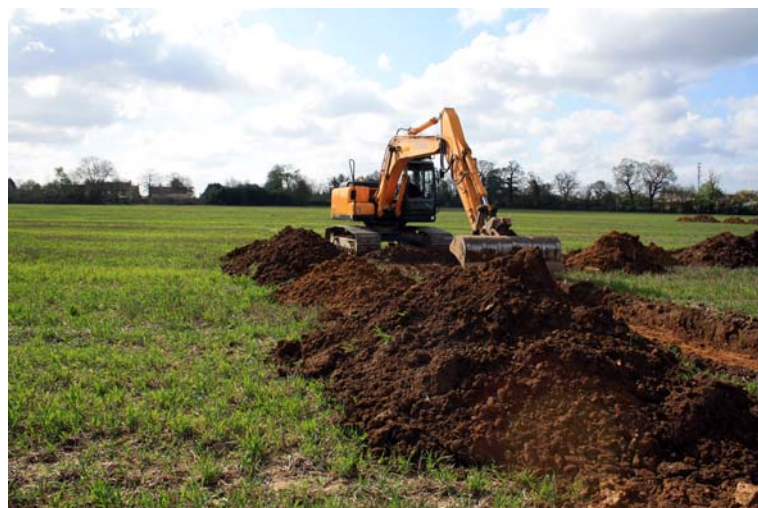
Plate 1. Machining the site
