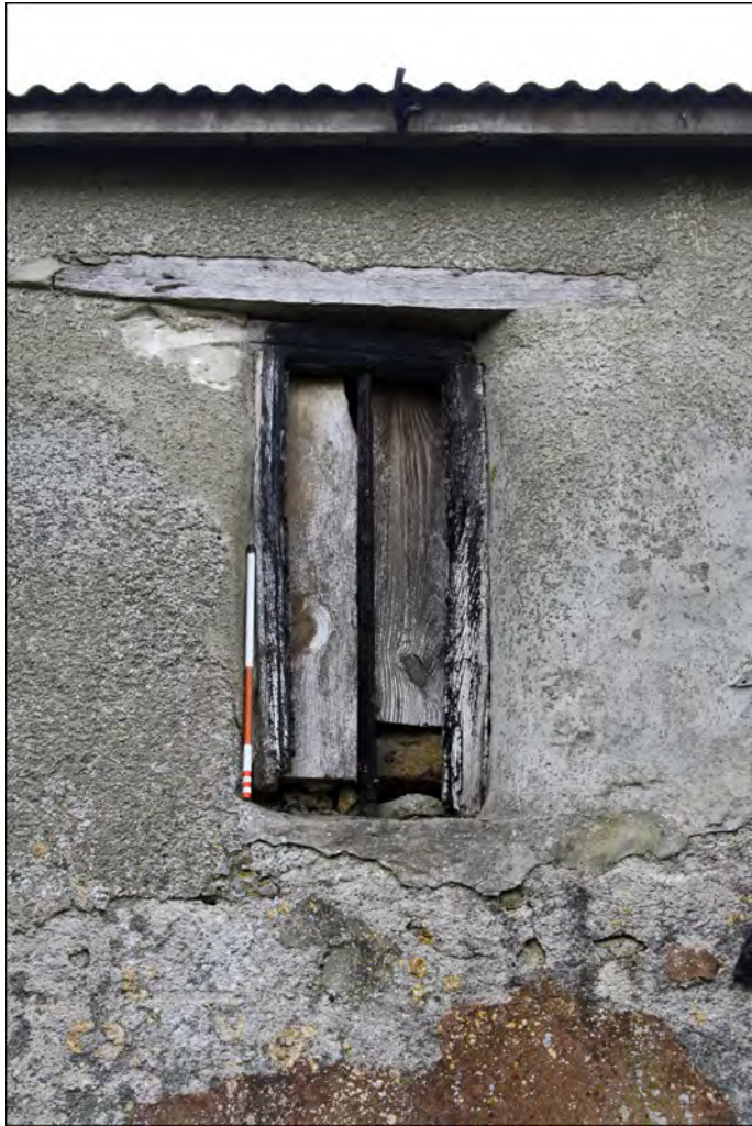
Plate 1. External view of window, 0.5m scale
