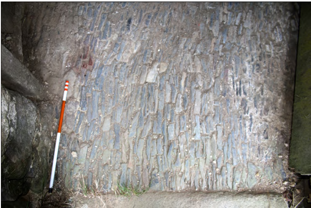
Plate 30. Cobbled floor to west, detail, 0.5m scale
