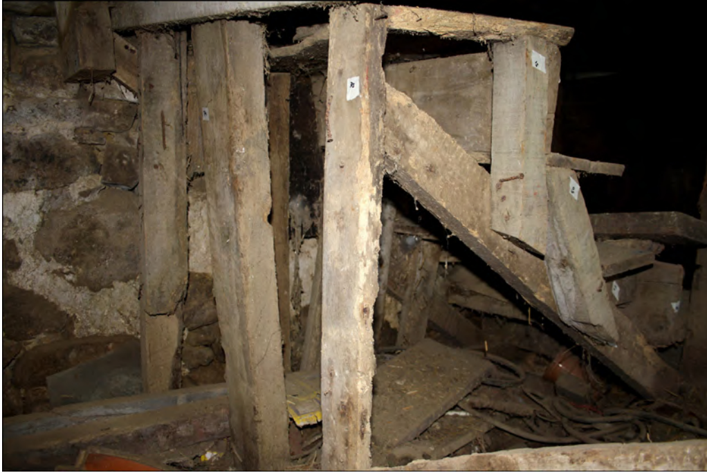
Plate 25. Below staircase, facing west
