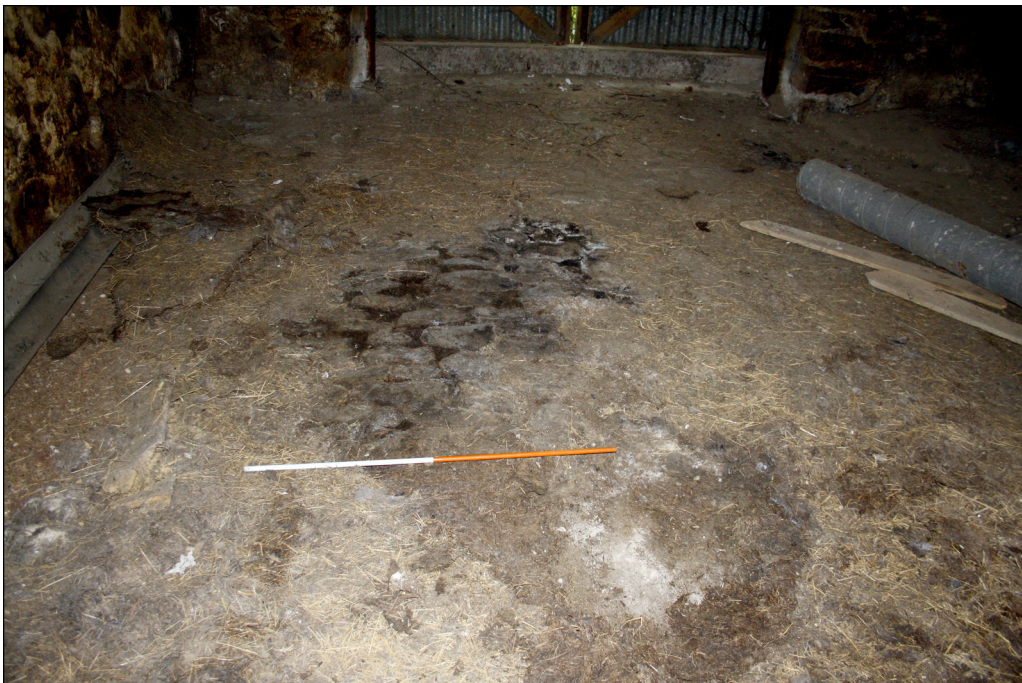
Plate 34. Cobbled floor at north end of barn, 1m scale
