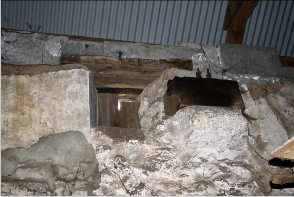
Plate 5. Internal view of window from below
