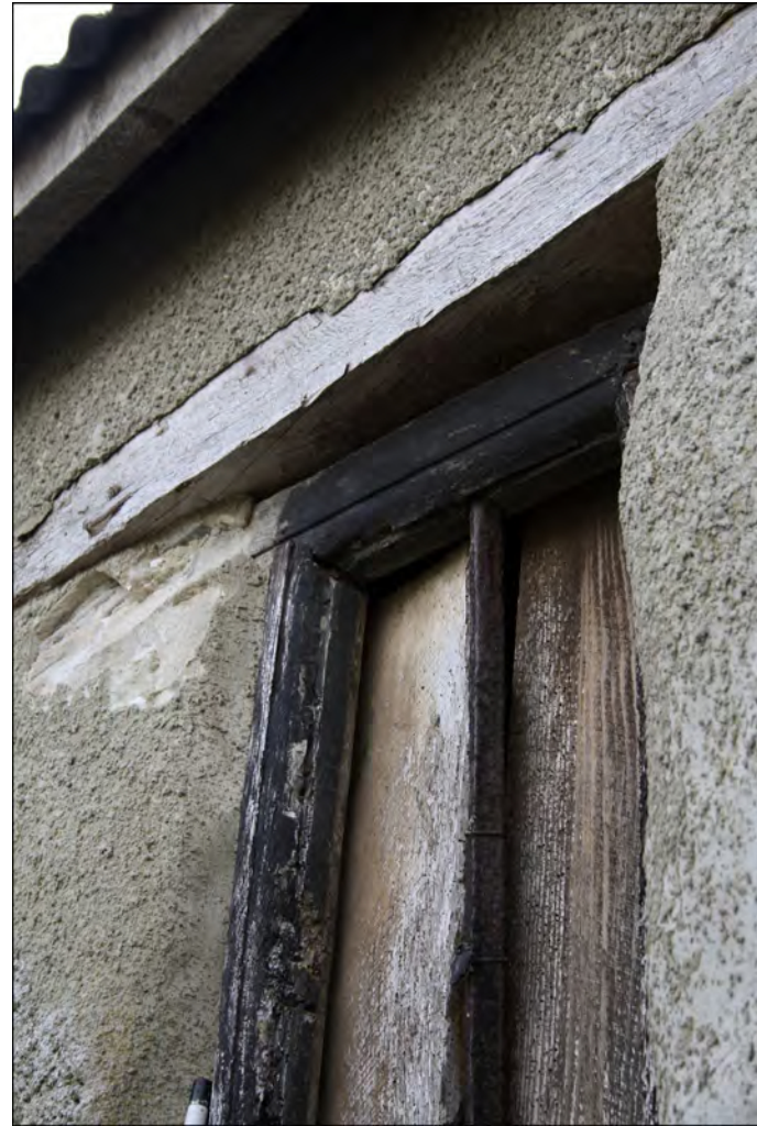
Plate 2. External view of window, detail
