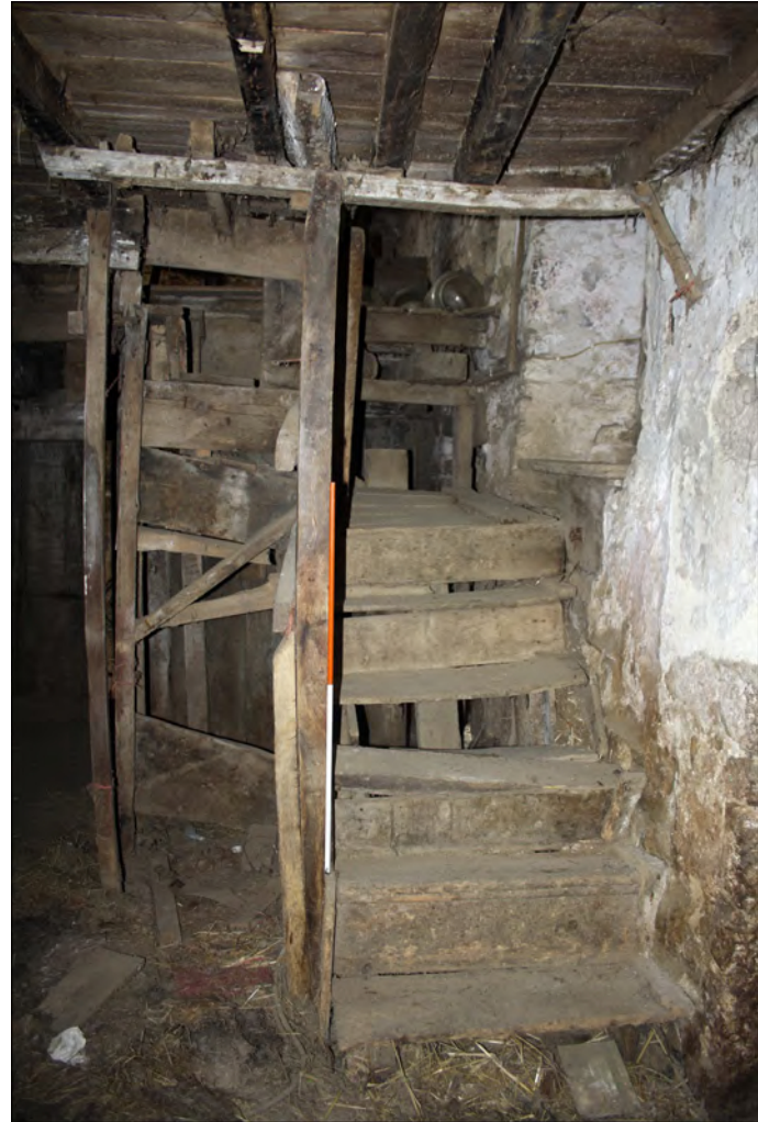
Plate 20. Stairs facing south, 1m scale
