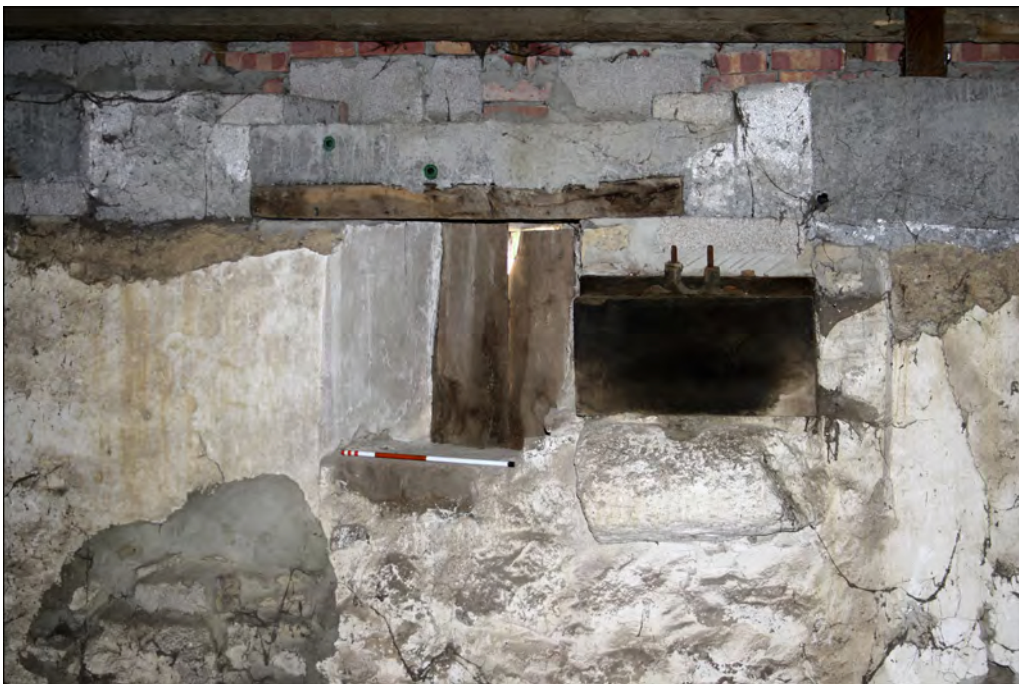
Plate 4. Internal view of window, facing east, 0.5m scale
