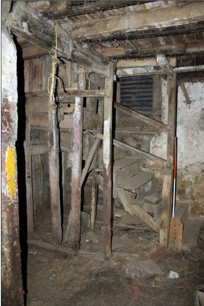
Plate 19. Stairs facing west, 1m scale
