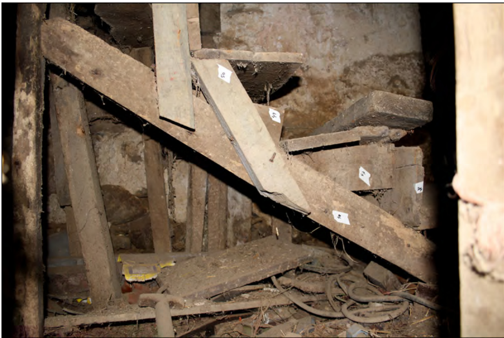
Plate 26. Below staircase, facing west
