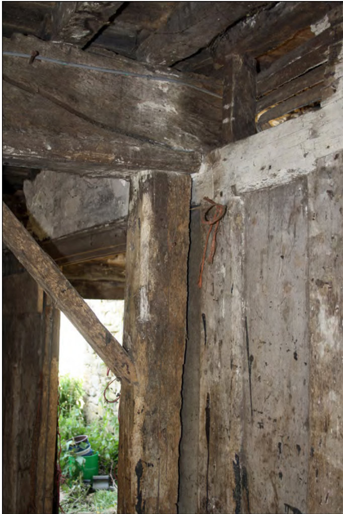
Plate 13. Ceiling timber above south screen
