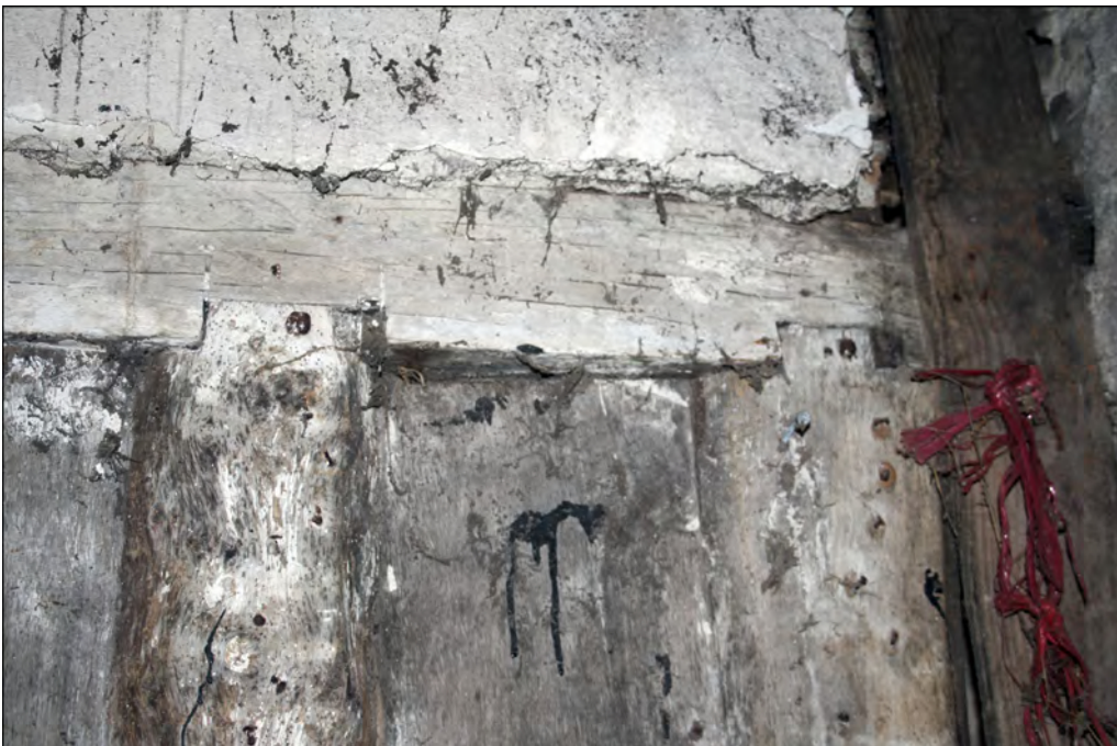
Plate 12. South screen, south elevation, east end
