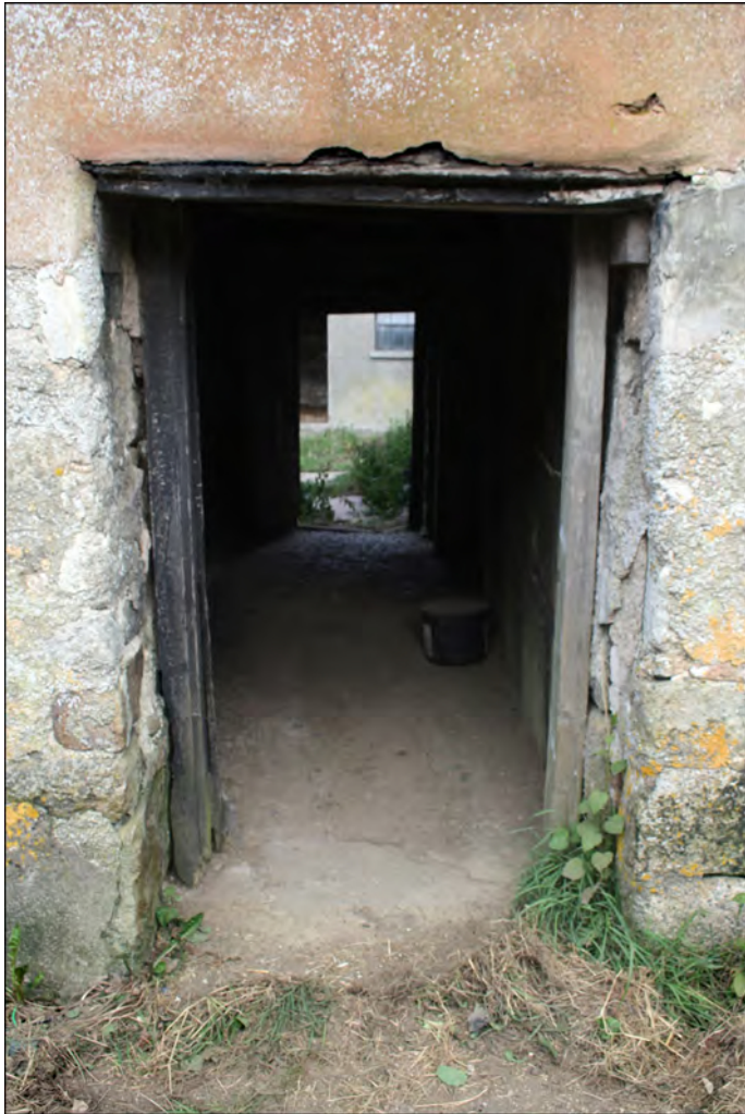
Plate 27. Cross passage from east door, facing west
