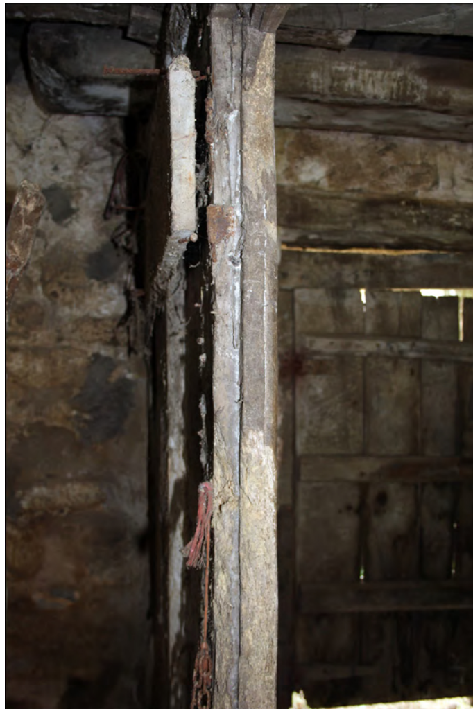
Plate 16. Width of southern screen, facing west
