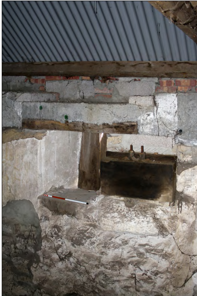
Plate 3. Internal view of window, facing east, 0.5m scale
