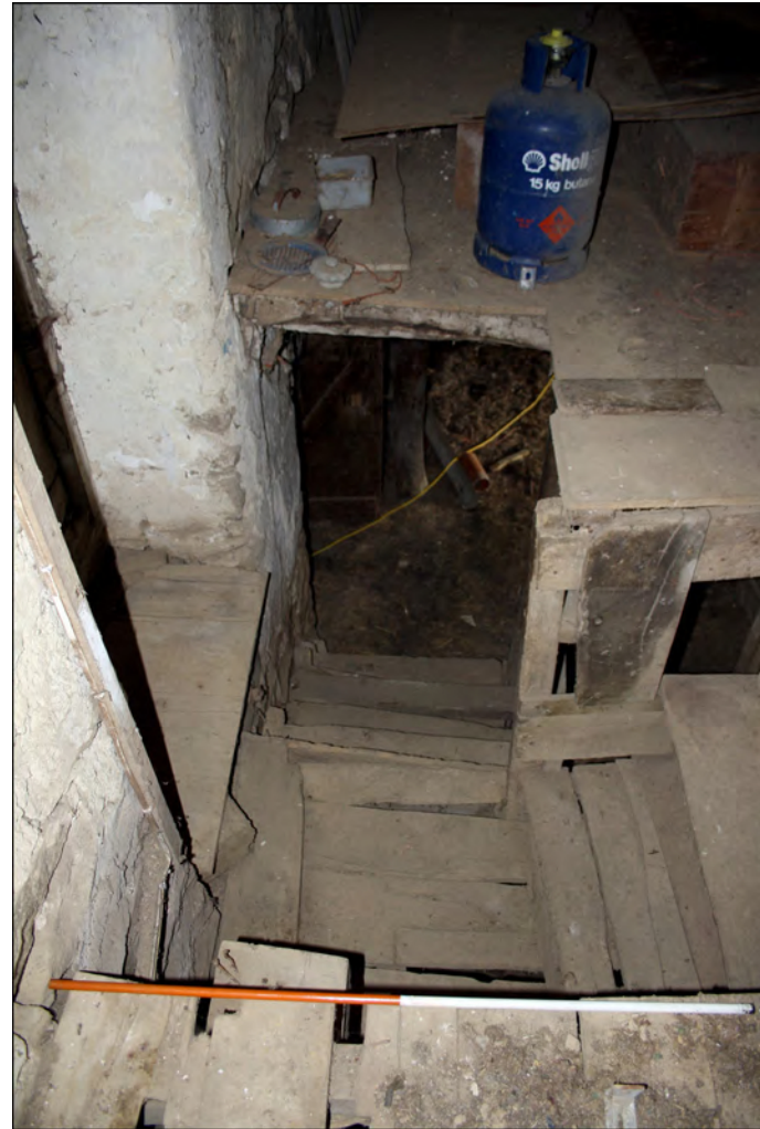
Plate 22. Stairs from above, facing north, 1m scale
