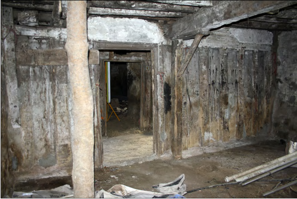
Plate 7. South screen, facing north
