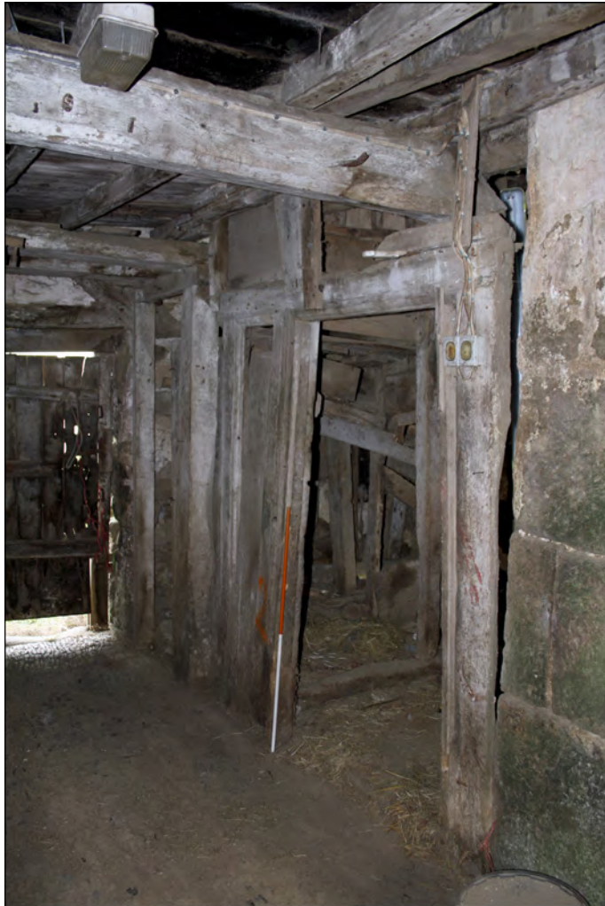
Plate 17. North screen passage, south elevation
