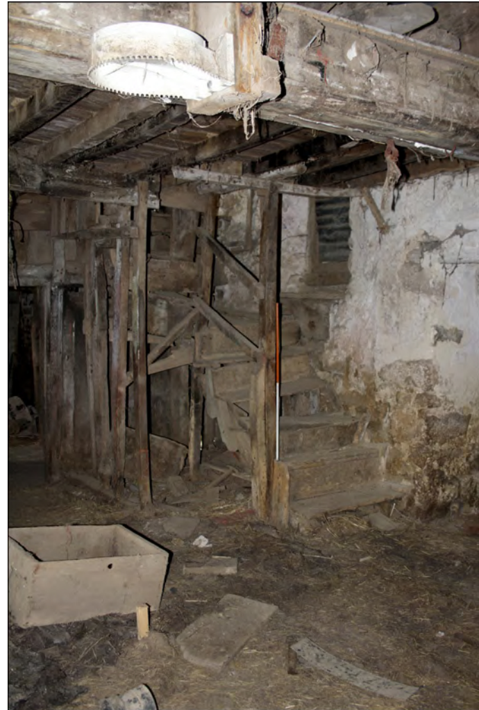
Plate 18. Staircase, facing south, 0.5m scale
