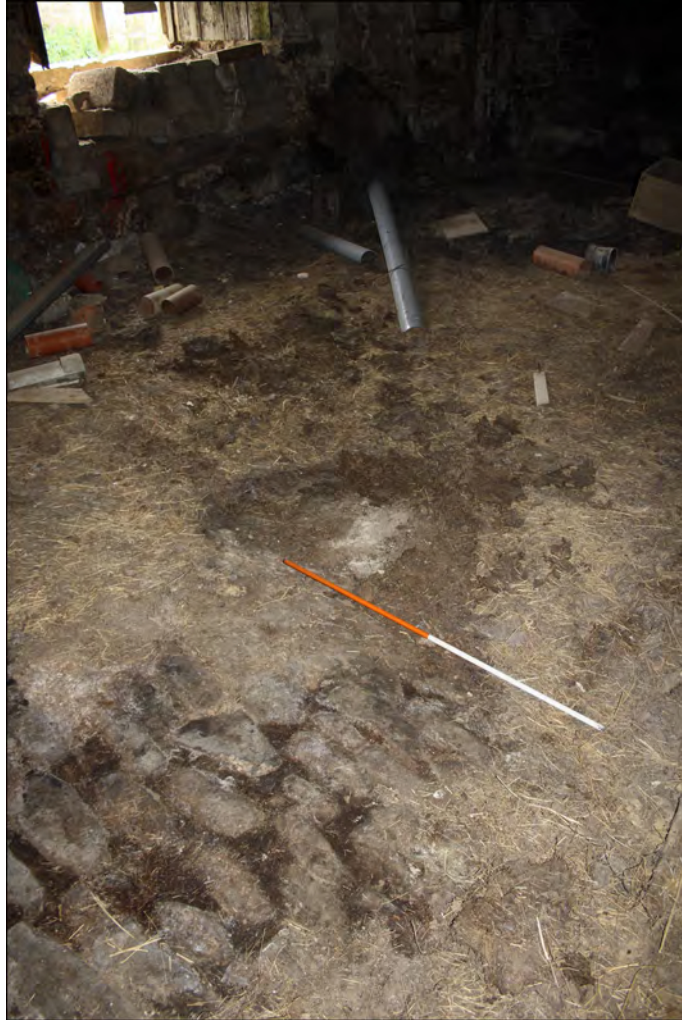
Plate 37. Cobbled floor at north end of barn, facing south-east, 1m scale
