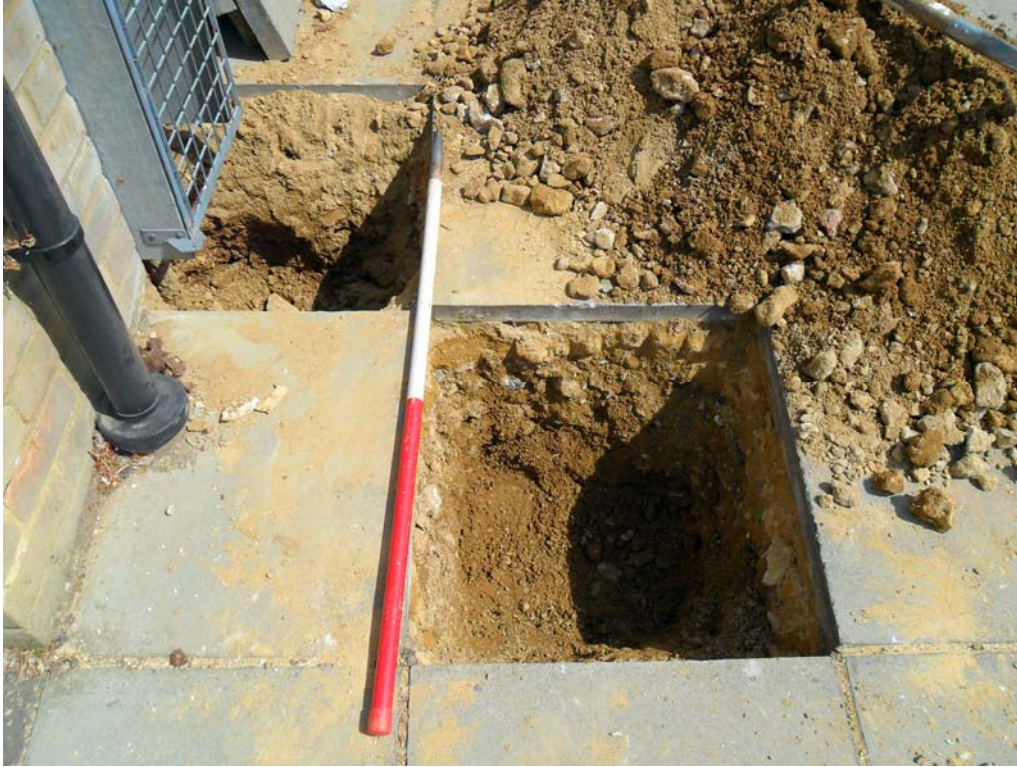
Plate 6. Connection to plant room
