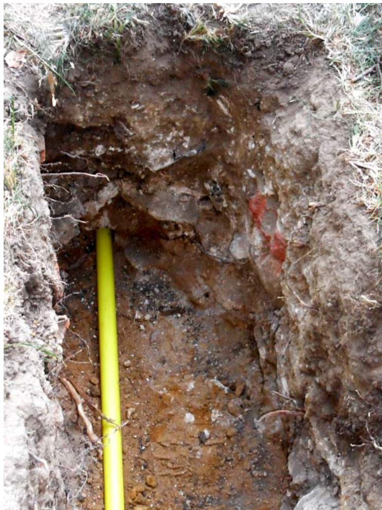
Plate 2. Close up section of Inspection pit 14
