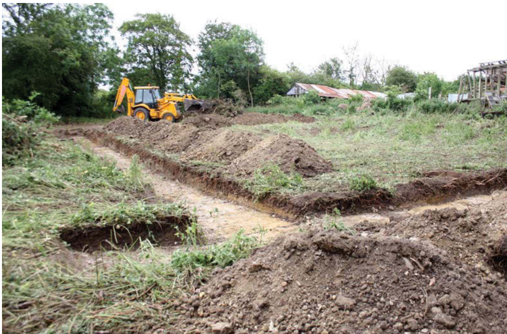
Plate1. Evaluation trenches, looking south
