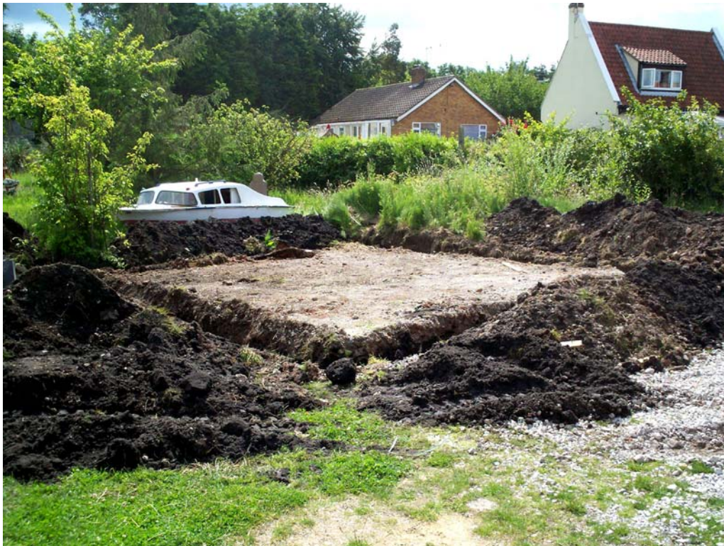
Plate 1: The site facing south-east
