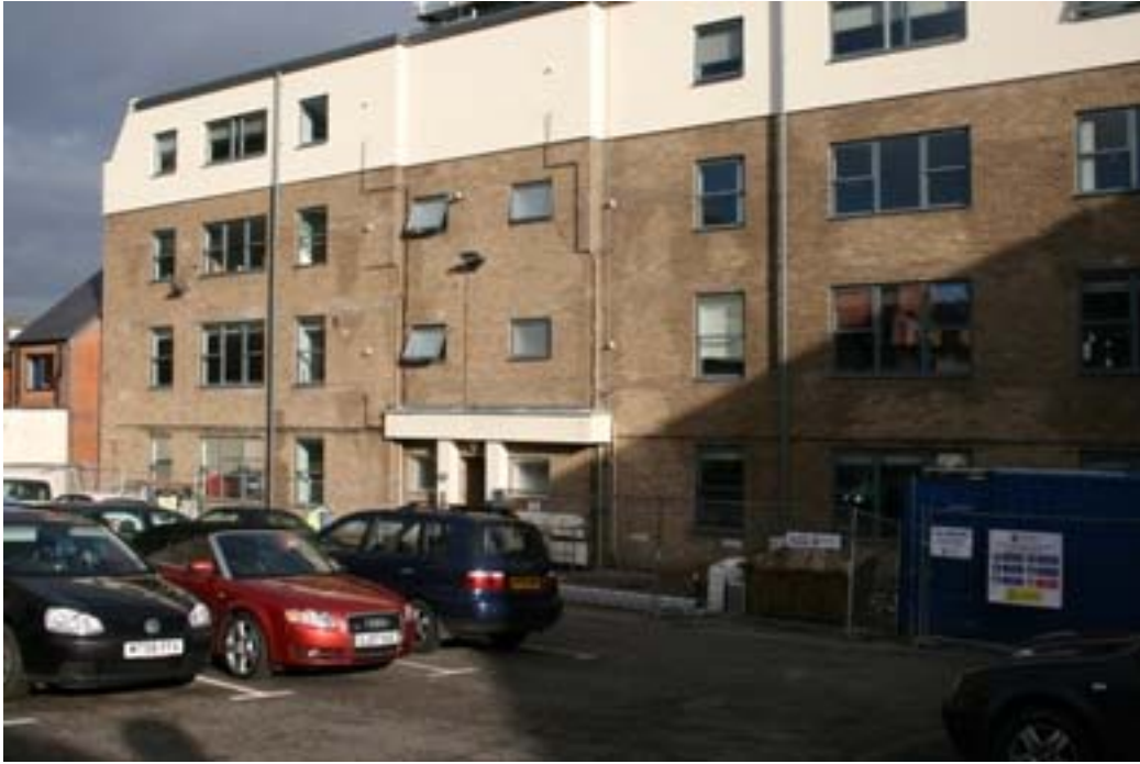
Plate 1. Development site, looking north-east
