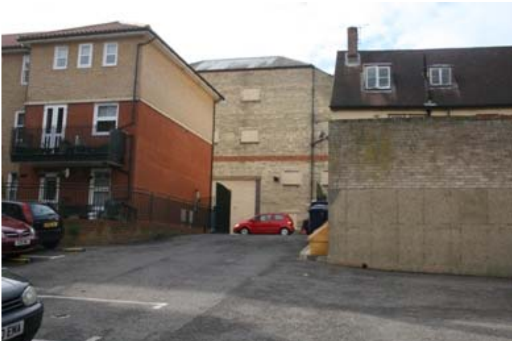
Plate 2. Development site, looking west
