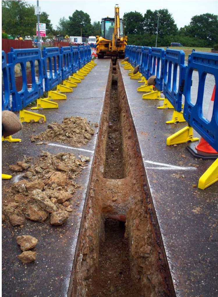
Plate 1: The pipe trench on Bridle Road
