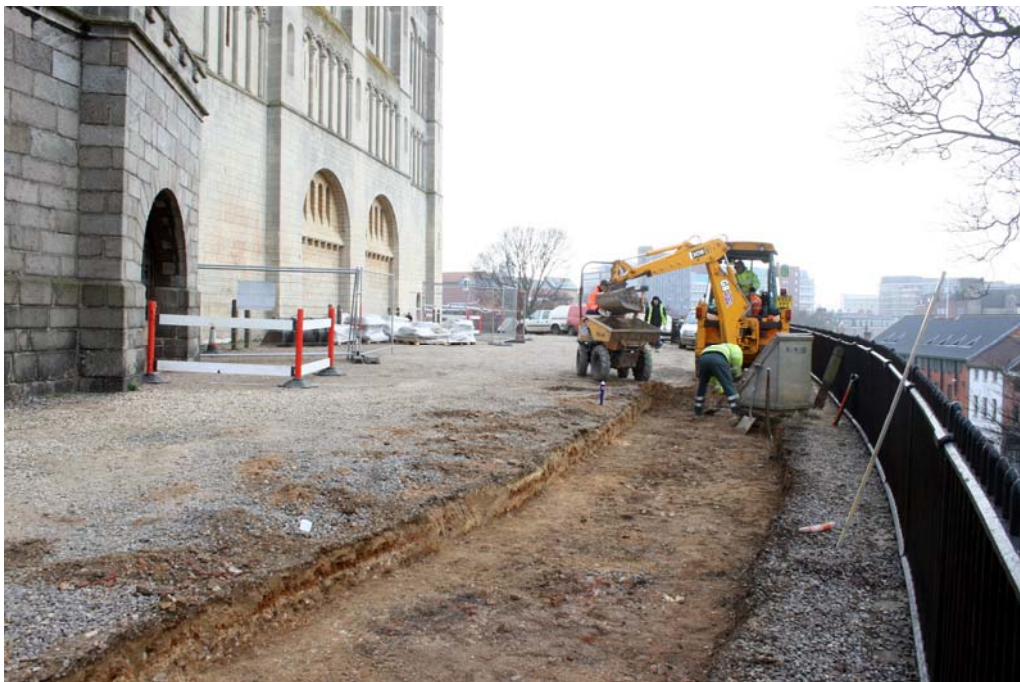
Plate 1. The site, looking south
