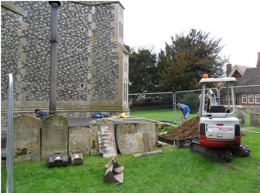
Plate 1. General view south-west showing the location of the boiler room.
