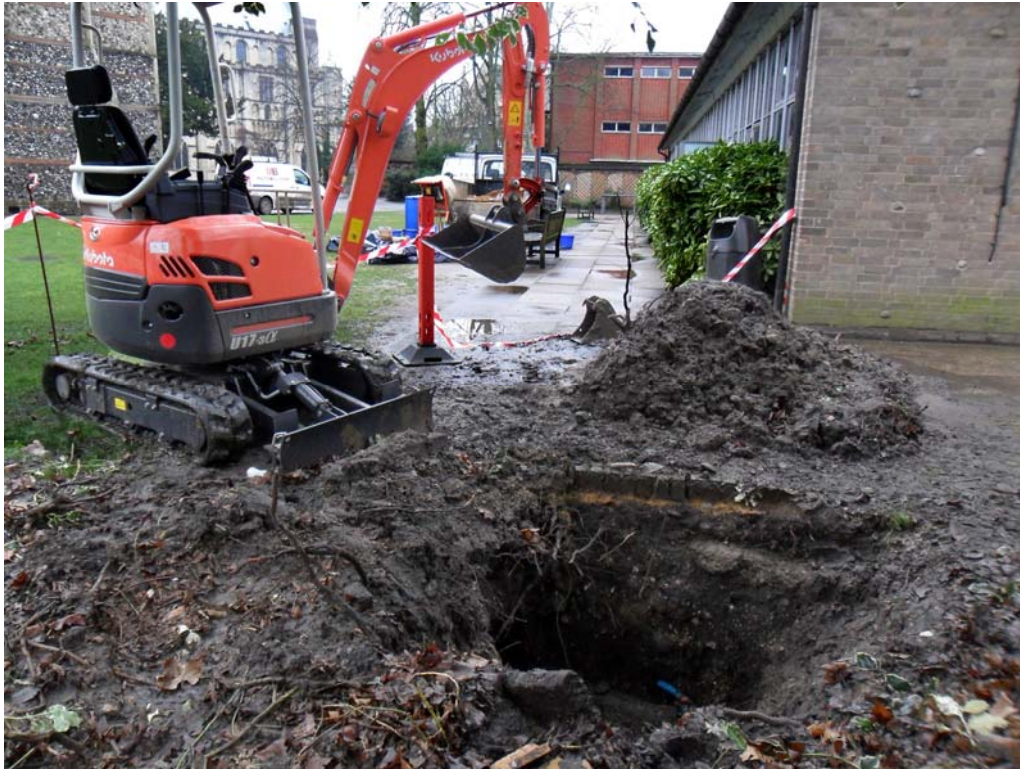
Plate 1. Excavation of the trench, looking south-west
