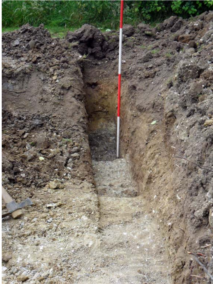
Plate 9 Extension of Trench 4
