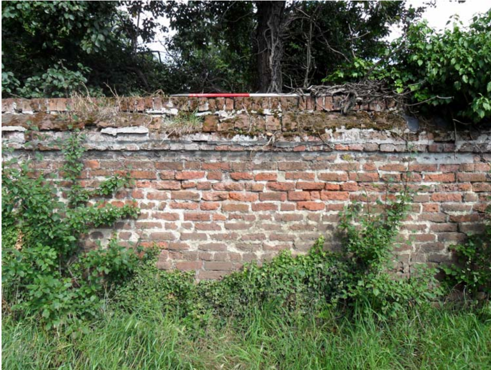
Plate 14. Typical example of decorative capping, external wall, looking east
