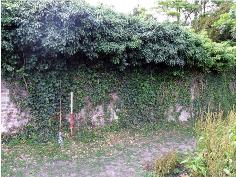
Plate 11. Internal section of wall to be removed, looking north-west
