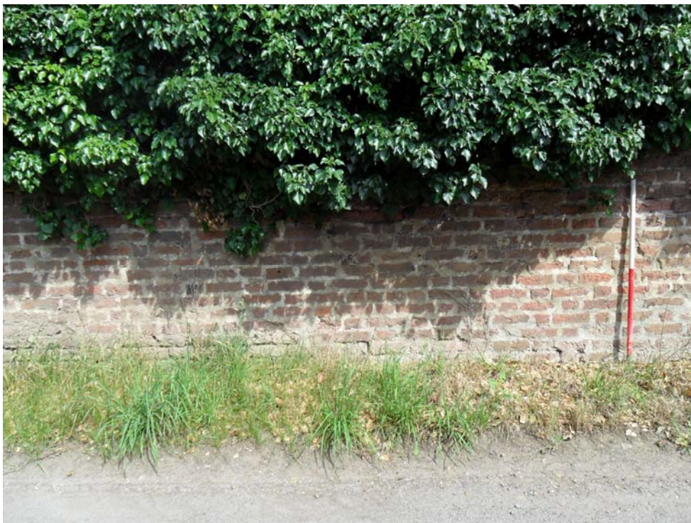
Plate 12. External section of wall to be removed, looking east
