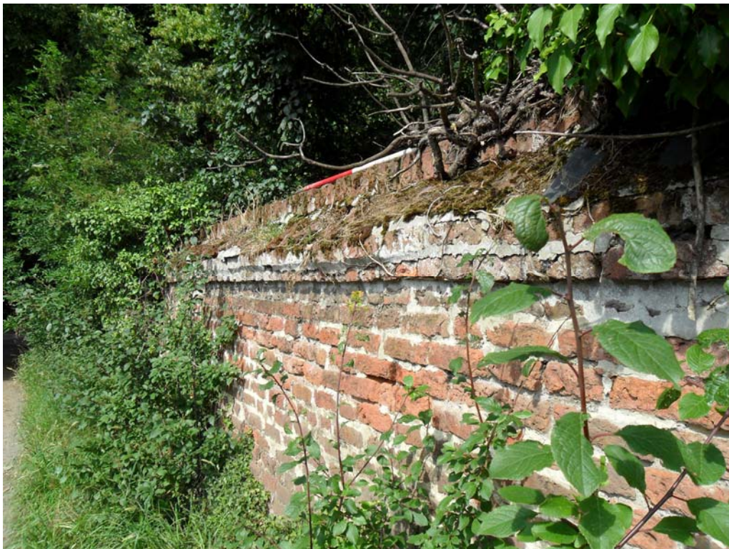
Plate 13. Typical example of decorative capping, external wall, looking north-east
