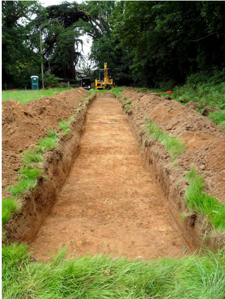
Plate 1. Trench following excavation, looking north-west (ditch [04] in foreground)
