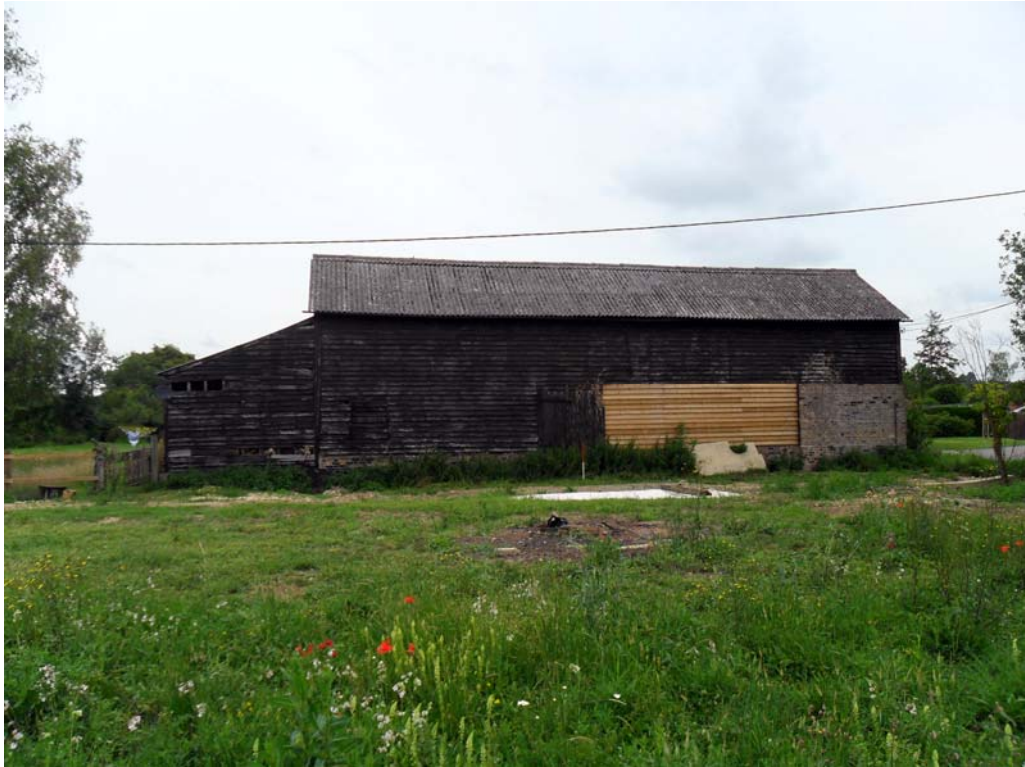
Plate 7. Building 1, exterior south side
