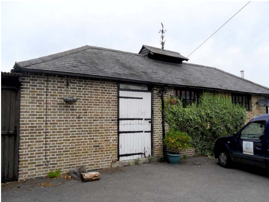
Plate 12. Building 2, exterior east side with blocked door behind van
