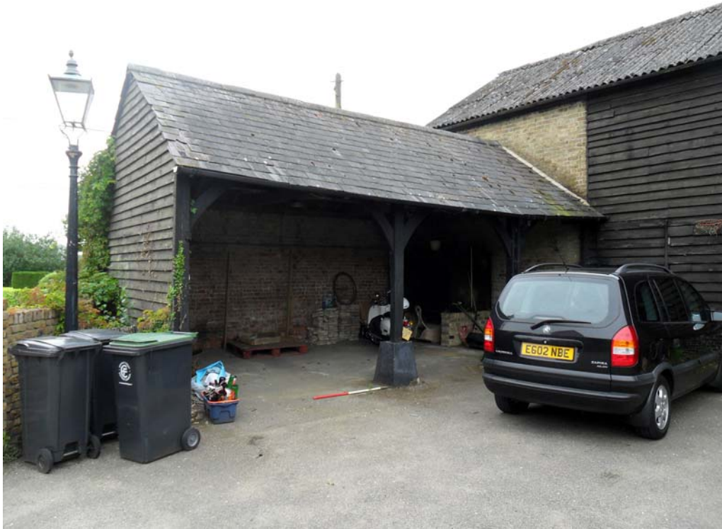
Plate 14. Building 3, exterior west face
