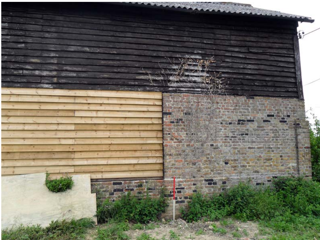
Plate 8. Building 1, rebuilt portion of south-east wall
