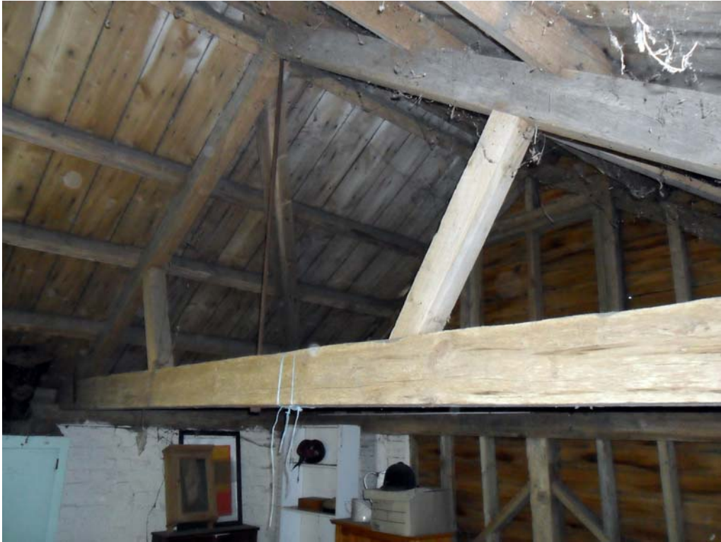
Plate 9. Building 1, example of roof truss, facing north-east
