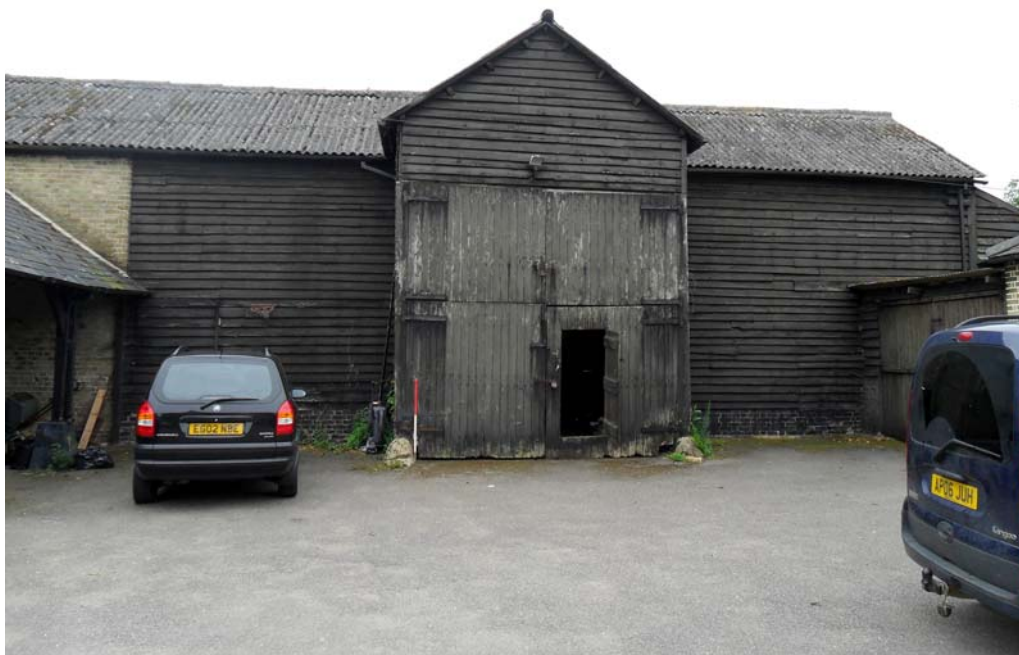
Plate 6. Building 1 exterior north side
