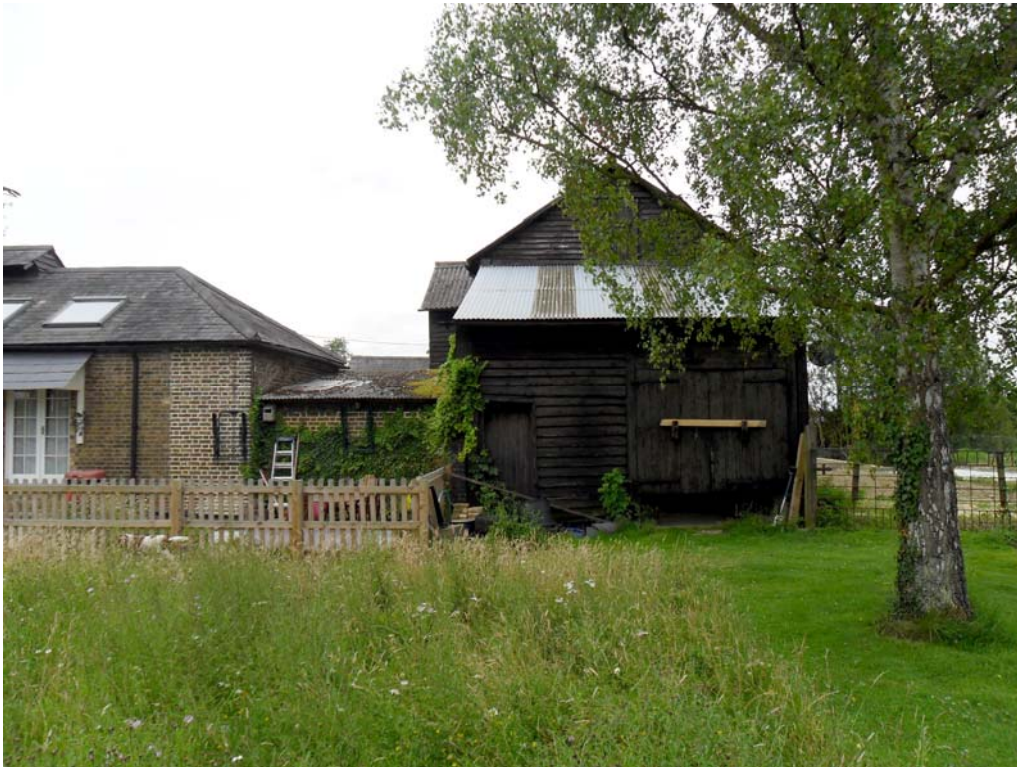
Plate 16. Building 5 (right), exterior west face, with Building 4 (centre), and Building 2 (left)
