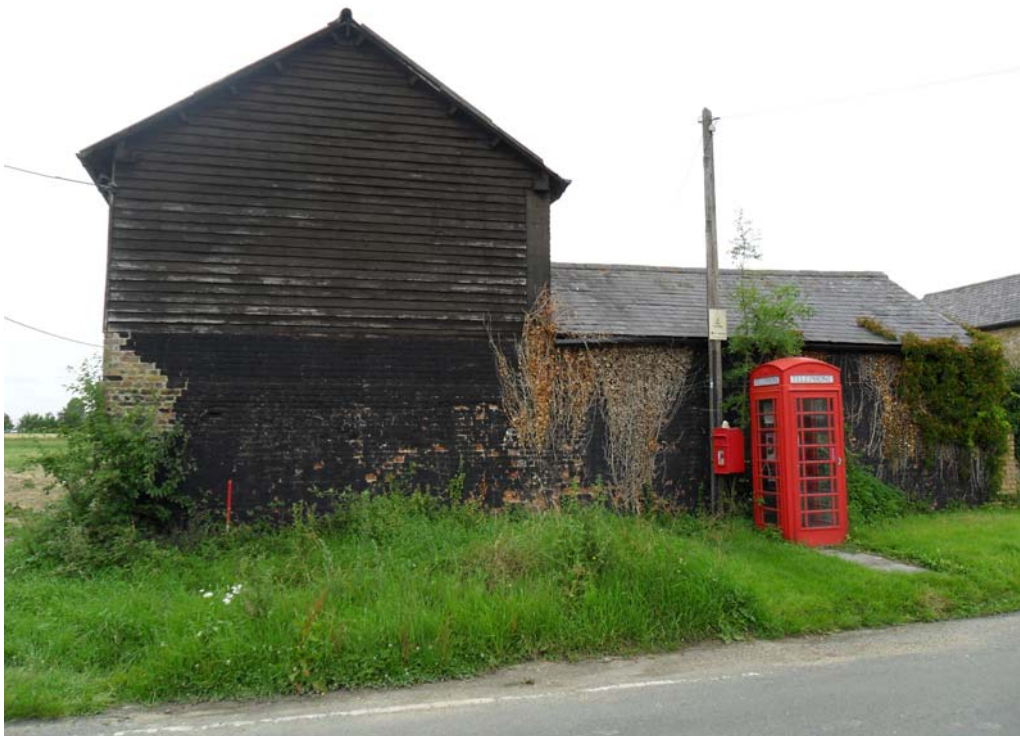
Plate 15. Building 3, exterior east face (right) with Building 1 to the left
