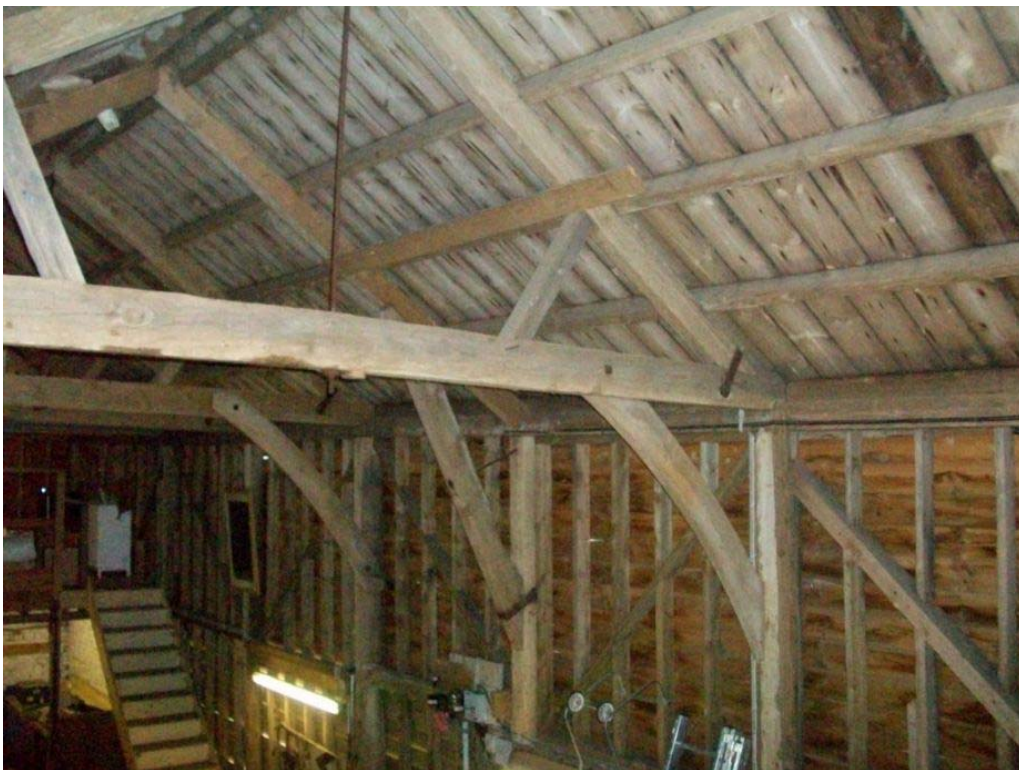
Plate 10. Building 1, roof detail, facing south-east
