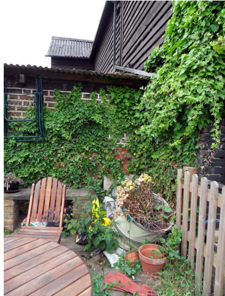
Plate 19: Building 5, exterior west face showing two possible phases of wall build
