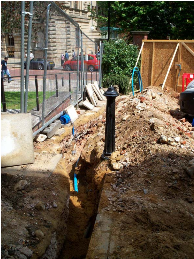
Plate 15. Service Trench facing north-east
