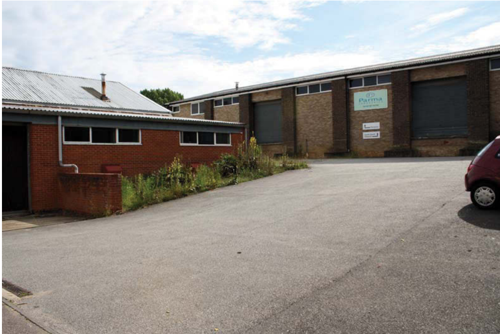
Plate 1. The site, from the High Street, looking east
