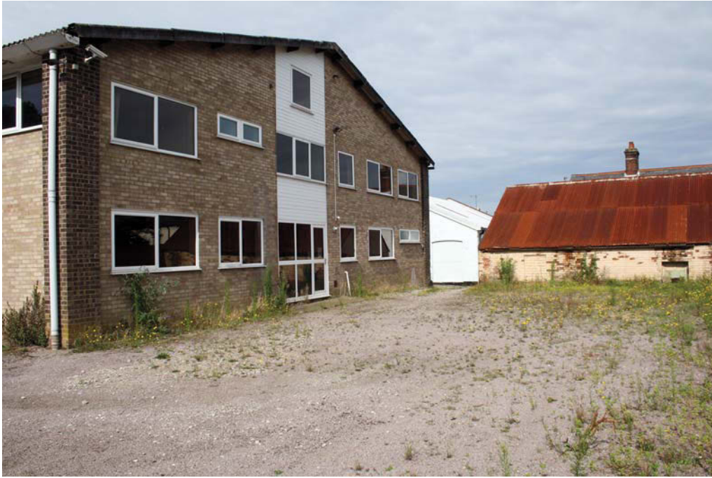
Plate 2. North-east elevation of modern factory building, with earlier outbuilding, looking west
