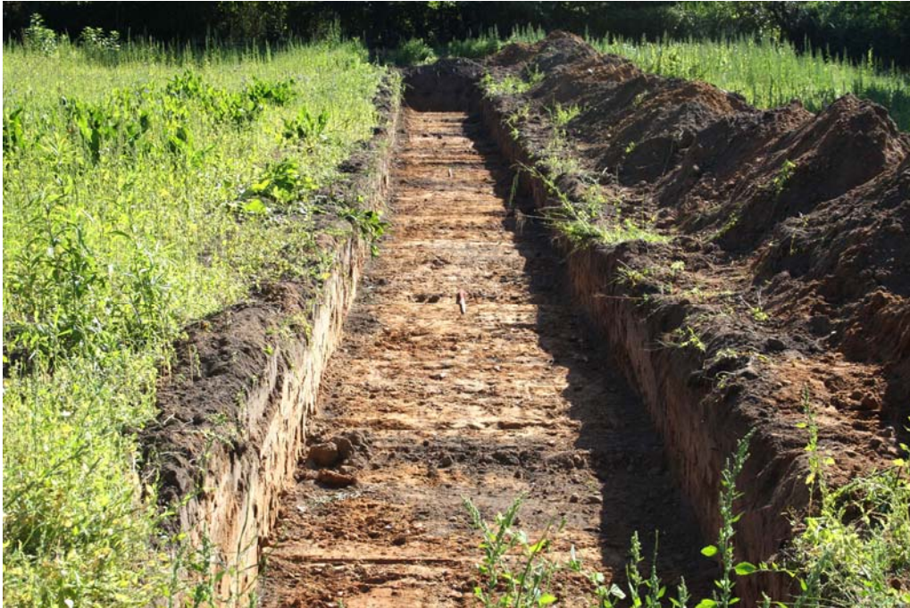
Plate 3. Trench 2, looking to the east along length of trench
