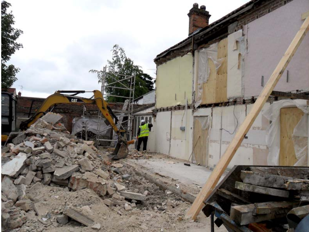
Plate 1. The demolition area to the rear of the house, looking south-east
