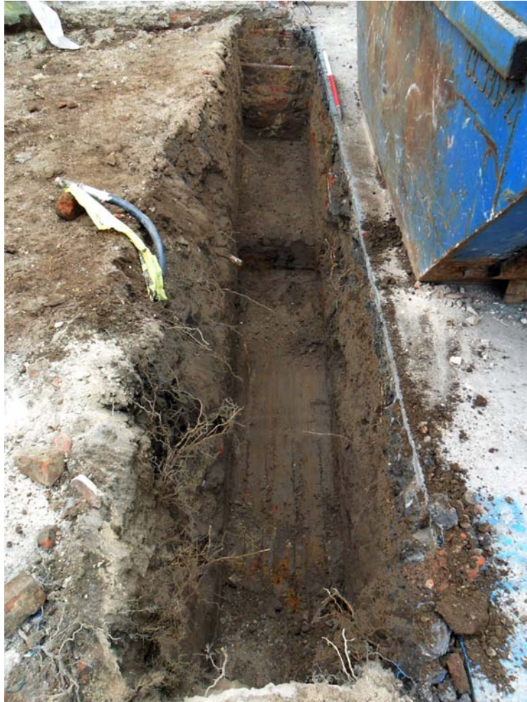
Plate 2. First trench, looking south
