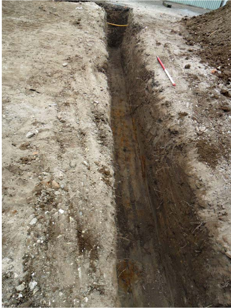
Plate 5. Third trench, looking north
