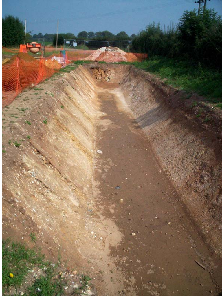
Plate 5. Infiltration Trench A, facing north
