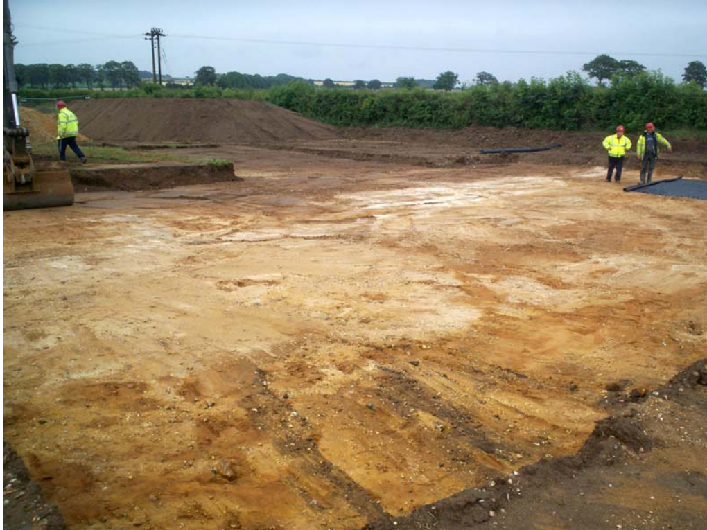
Plate 3. Initial strip of the Workshop area, facing south-east showing subsoil and topsoil layers
