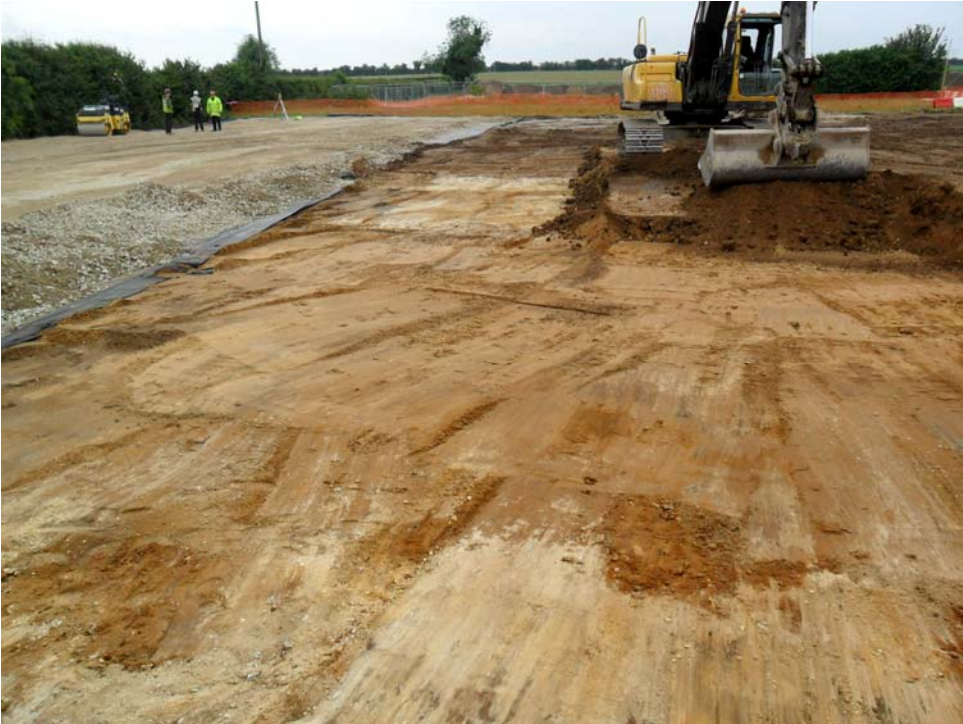
Plate 2. Initial strip of the General Store, facing north
