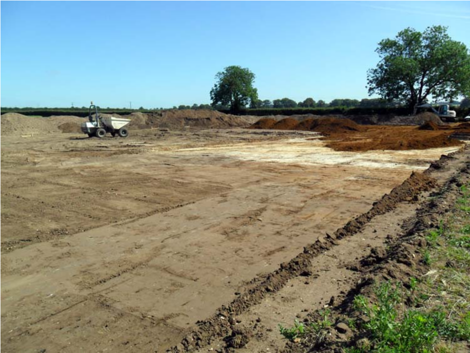
Plate 1. Initial strip of the Potato Store, facing south-east
