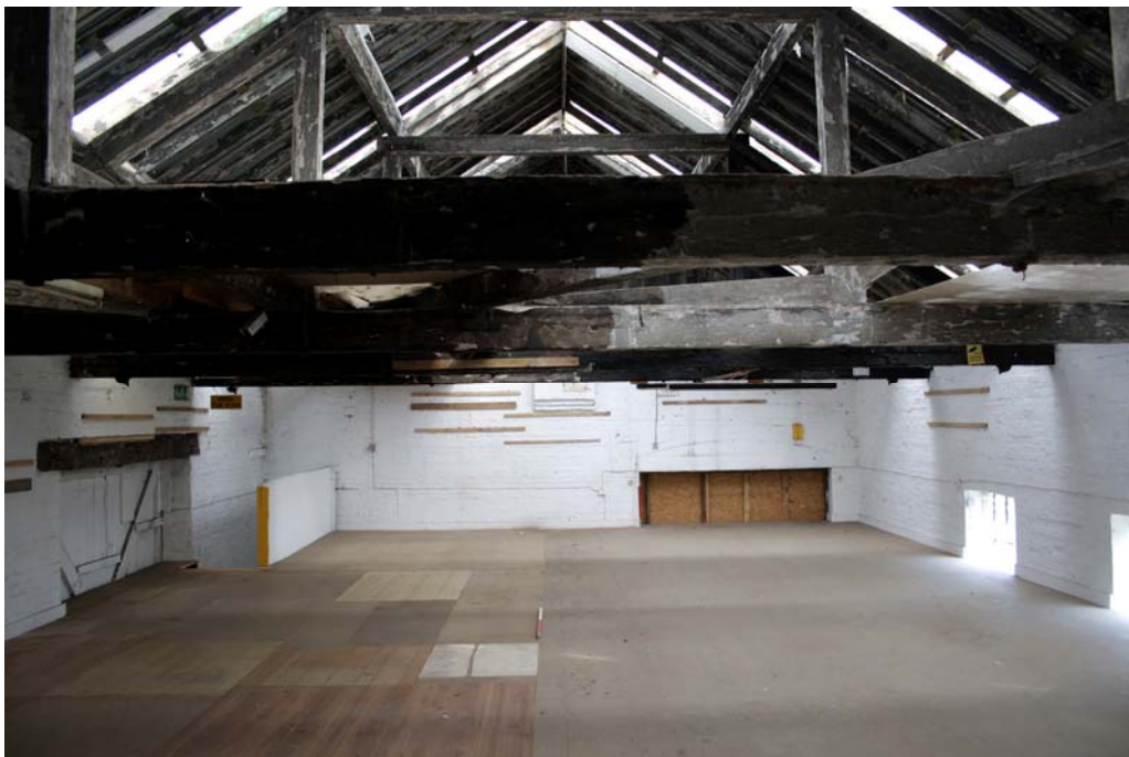
Plate 6. General view north-east of upper floor of goods shed interior
