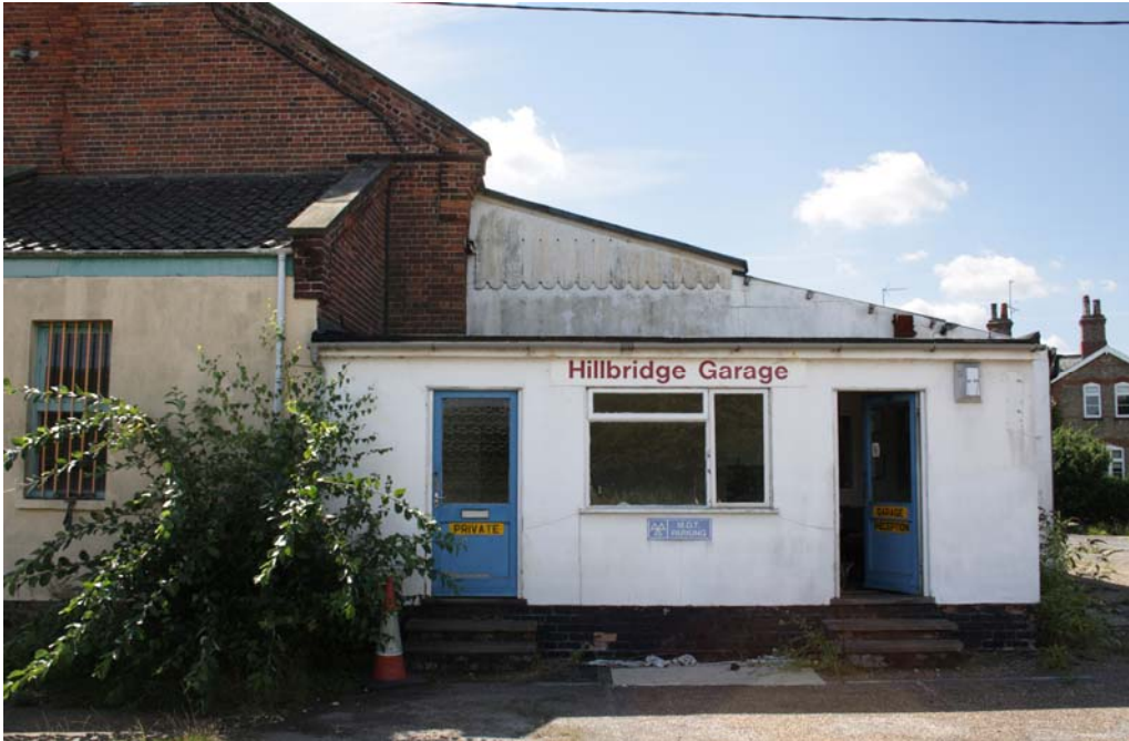
Plate 2. The scalloped timber side panel of the loading bay canopy
