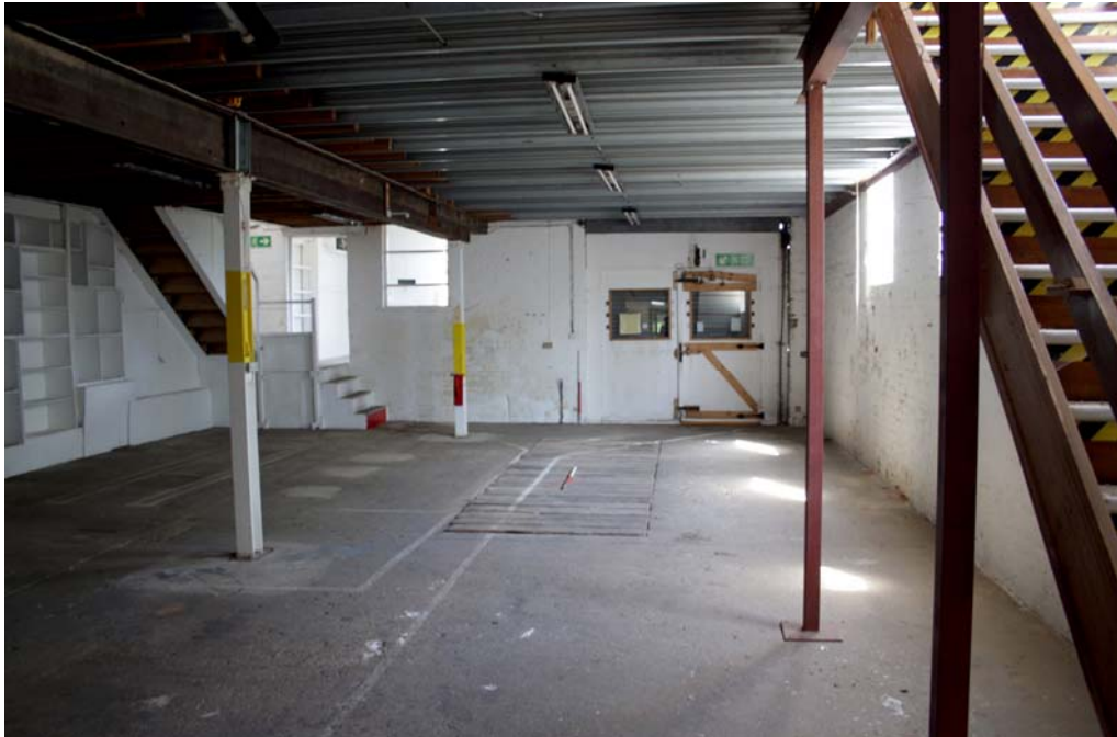
Plate 4. General view north-west of goods shed interior
