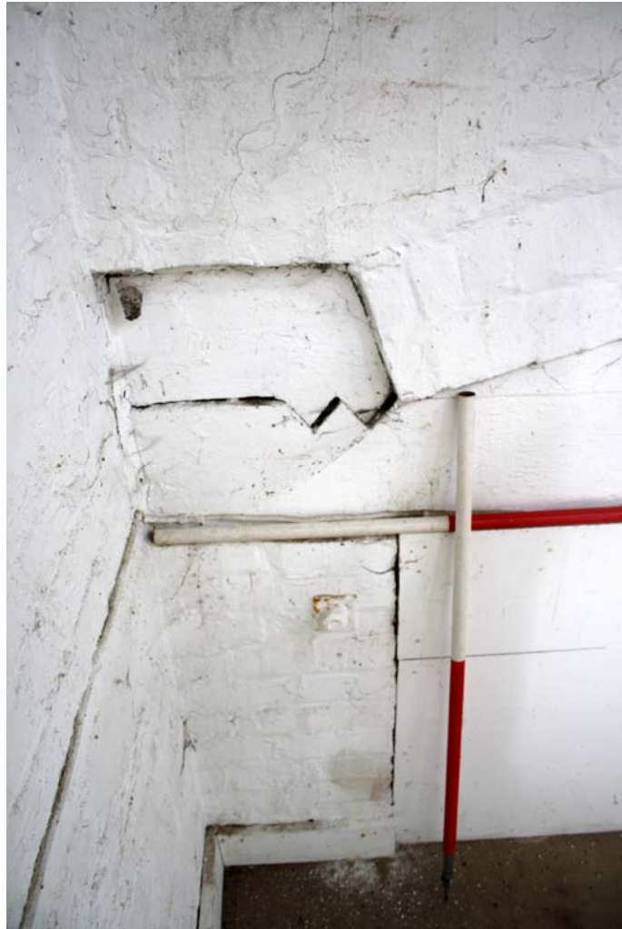
Plate 7. Detail of 'shark-tooth' joint above railway door
