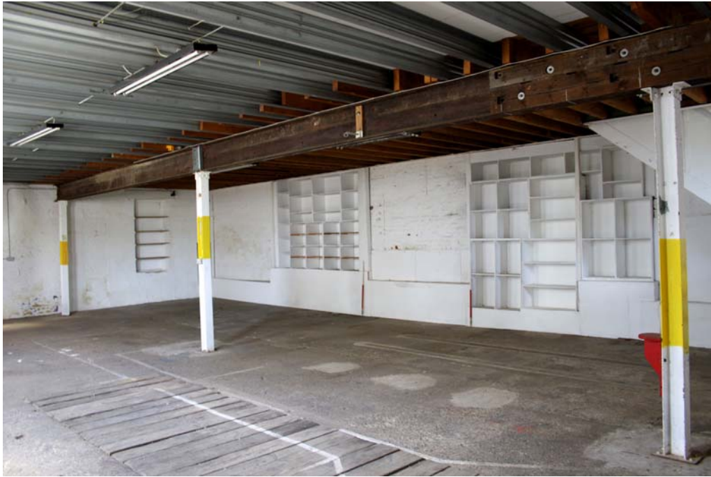
Plate 9 Upper section of loading doors
