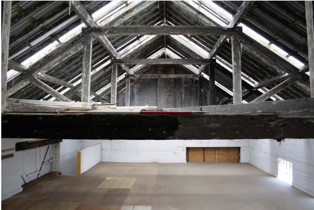
Plate 12 General view of roof structure
