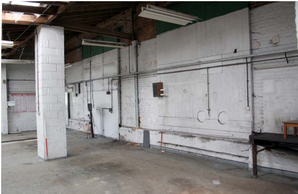
Plate 10 Exterior of loading doors in former loading bay
