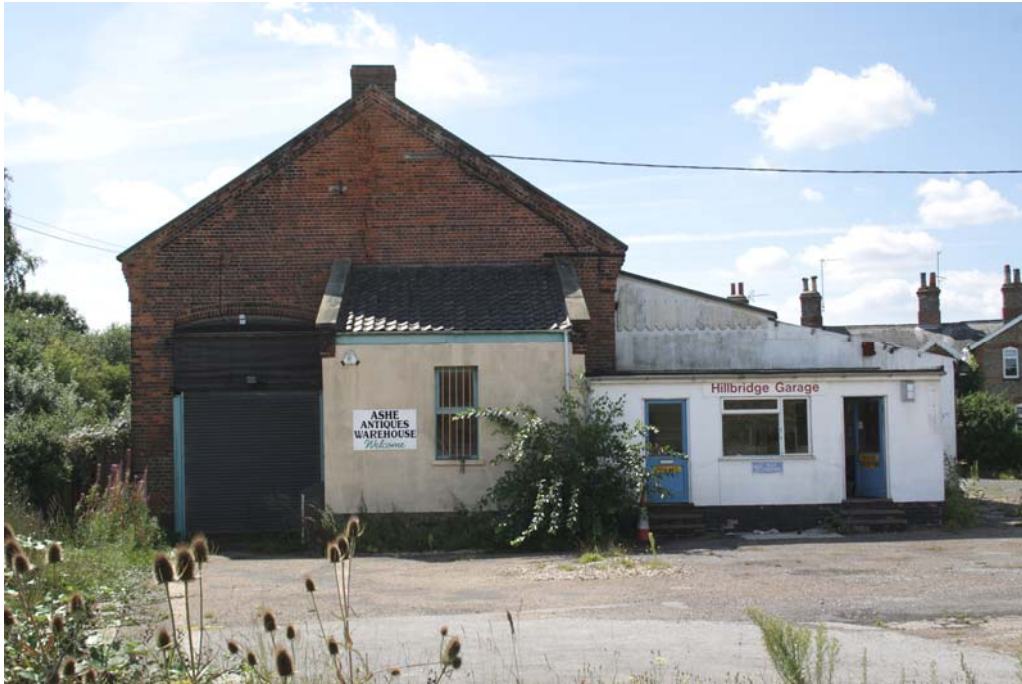
Plate 5. North-east gable wall showing former railway door
