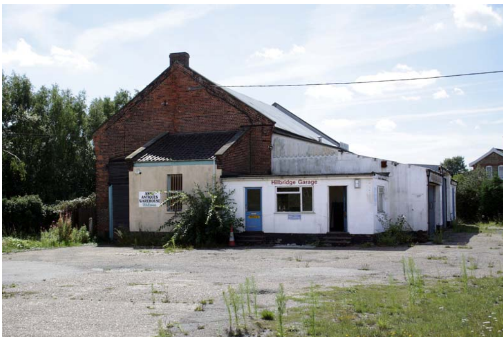
Plate 1. General view south-east of goods shed
