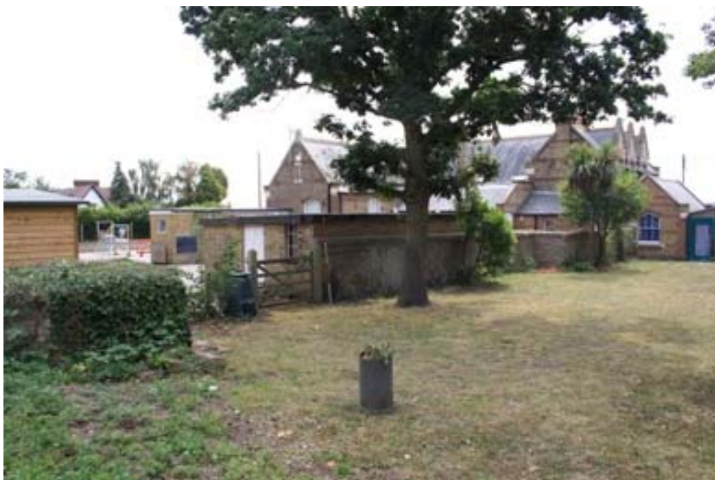
Plate 2. General view south-east of the air raid shelter
