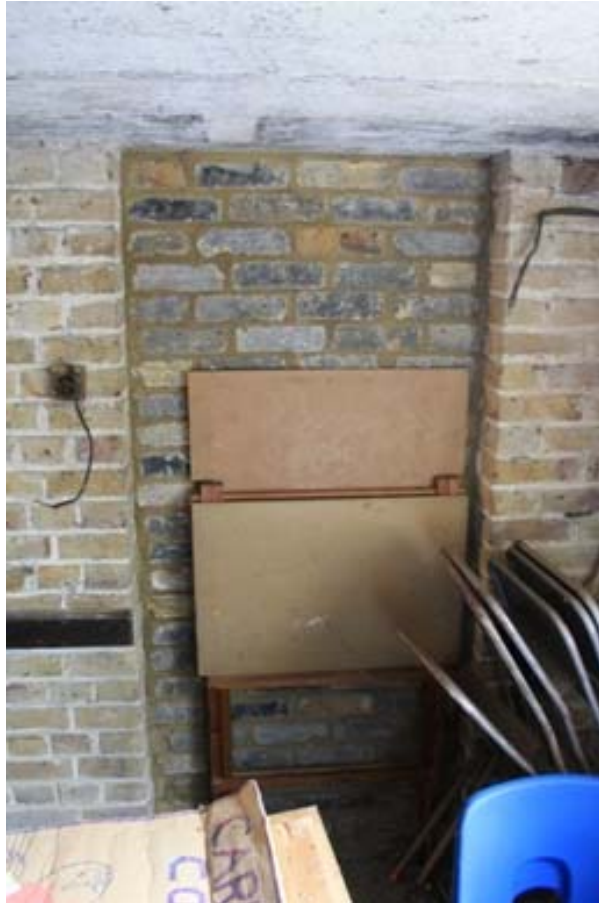
Plate 6. Blocked doorway between rooms 2 and 4 and the remains of a Bakelite switch
