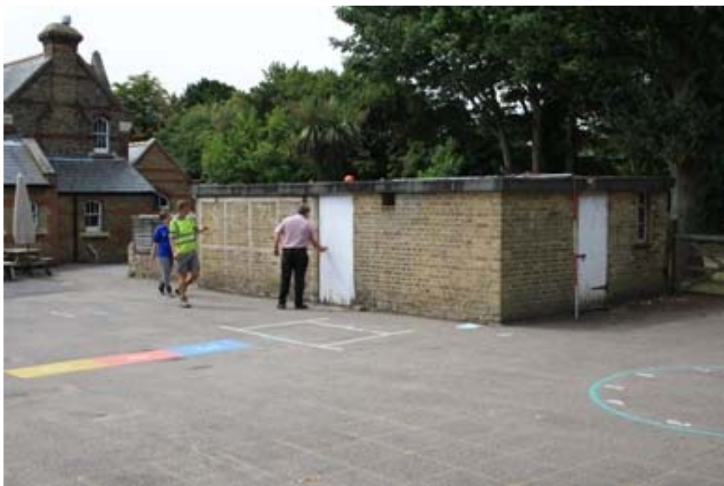
Plate 1. General view south-west of the air raid shelter
