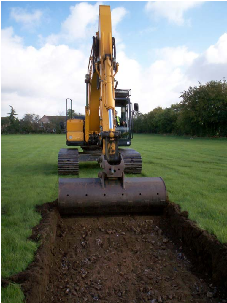
Plate 1. Machining one of the trenches
