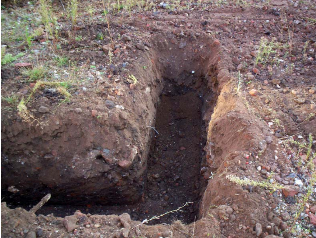
Plate 2. Section of foundation trench looking east, 1m scale
