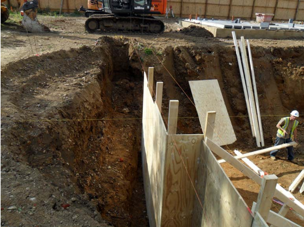
Plate 2. Area of disturbance from the old pub's cellar
