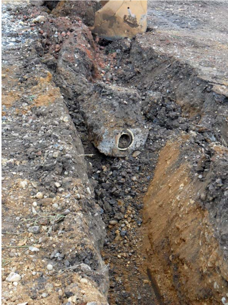
Plate 5. Modern services in trenches for Plots 16-19
